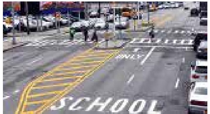
61st Street / Northern Boulevard: Vision Zero projects on this street include two new pedestrian islands, simplified vehicle movements, increased visibility for drivers, and a signal modification that gives pedestrians a "head start"
