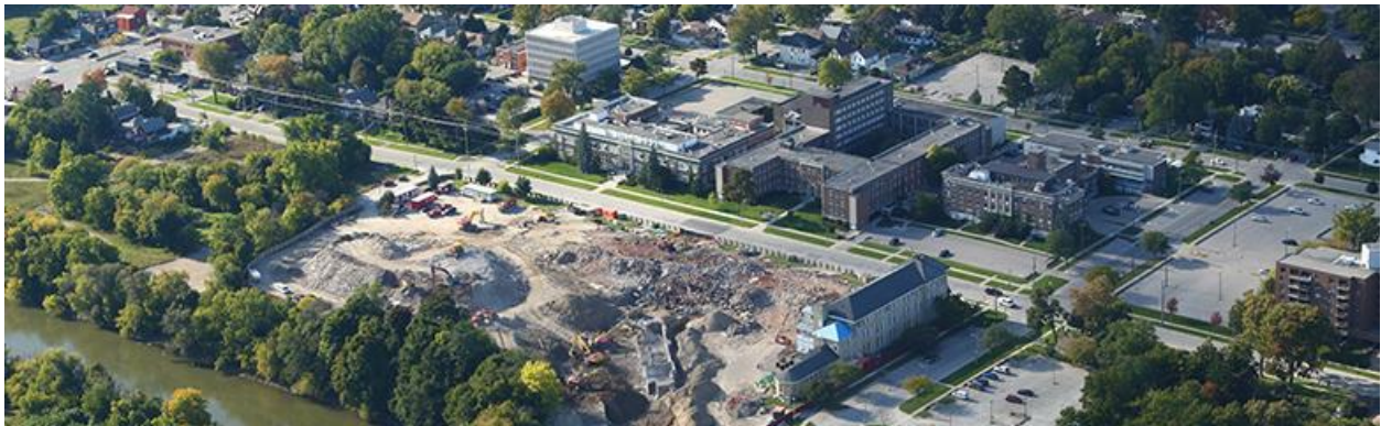
Image 3: Old Victoria Hospital lands following the Phase 1 demolition process in 2014.
