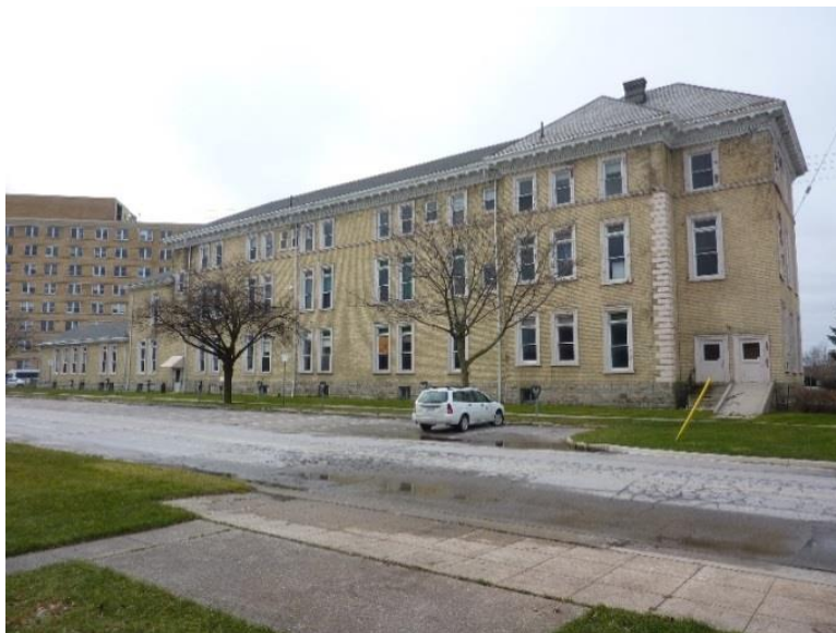
Image 4: Colborne Building (circa 1899 with later additions).
