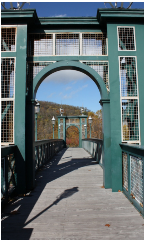
An example of a pedestrian bridge.
