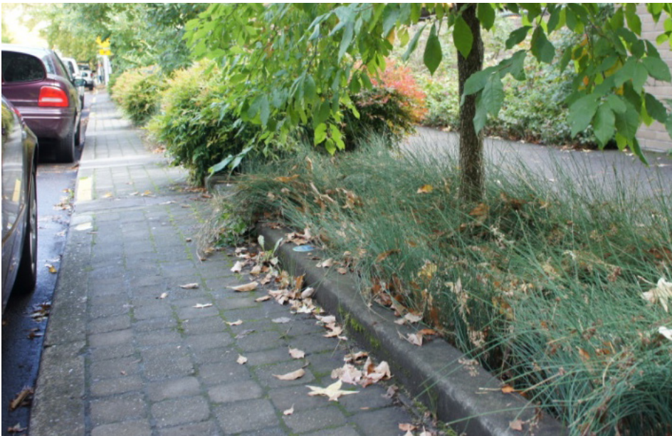
Examples of alternative stormwater management systems that slow the rainwater intake into the system, relieving pressure from the system during large storm events.
