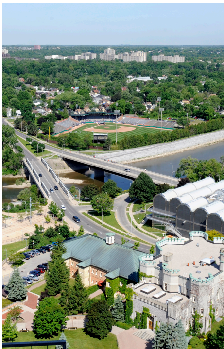
Looking west from the downtown at Kensington Bridge.
