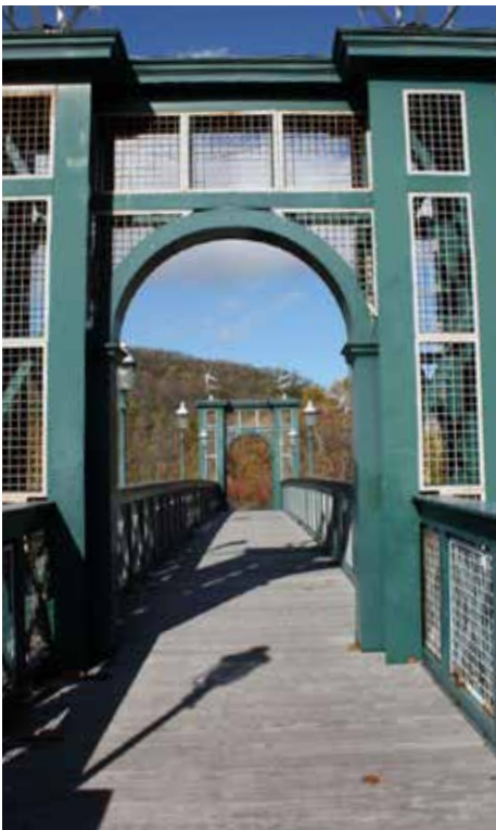
An example of a pedestrian bridge.
