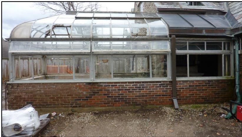
Rear – Greenhouse from north
