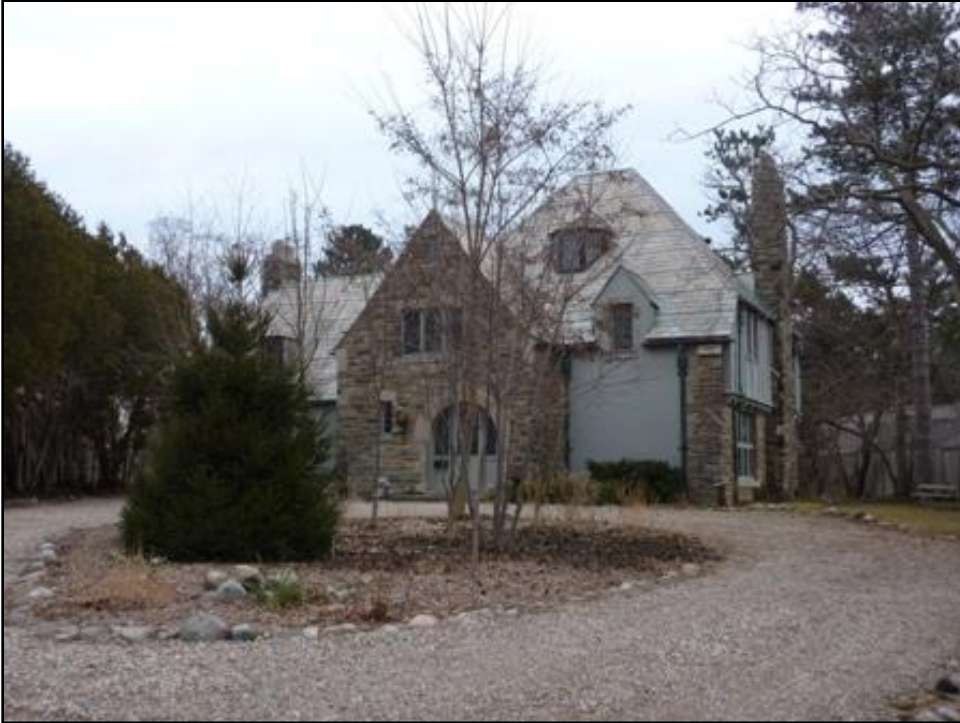
Front façade-facing Richmond Street
