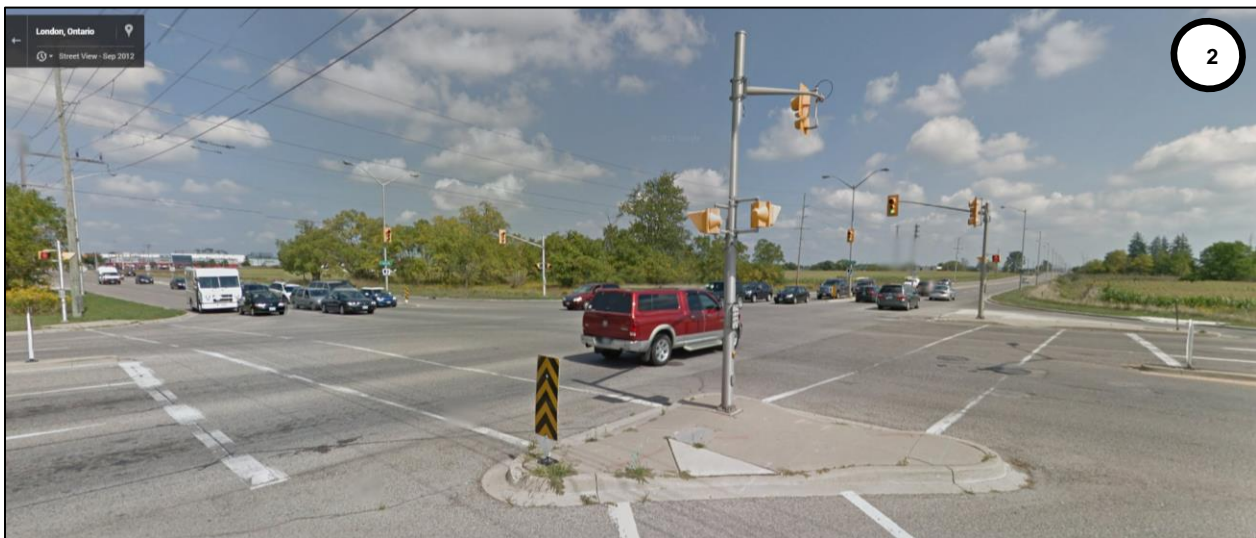
Street View: Looking northeast toward site from Exeter Road and Wonderland Road South.
