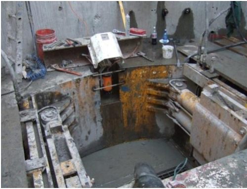
Figure 3: Jacking wall and lazer
