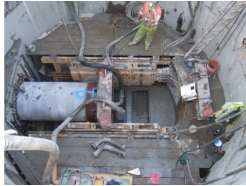
Figure 4: Working platforms in shaft
