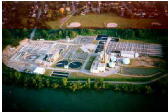
Greenway Water Treatment Plant
