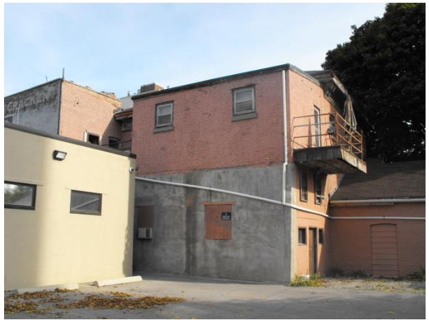
Image 3: West elevation showing 1880s structure and 1922 structure (October 24, 2014)
