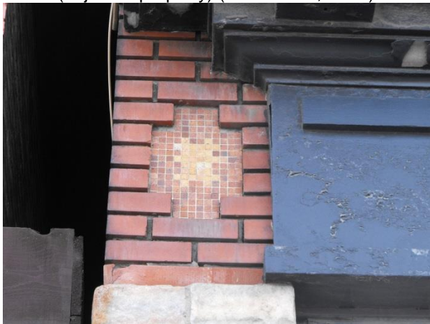
Image 6: Mosaic tile detailing flanking the cornice (October 24, 2014)
