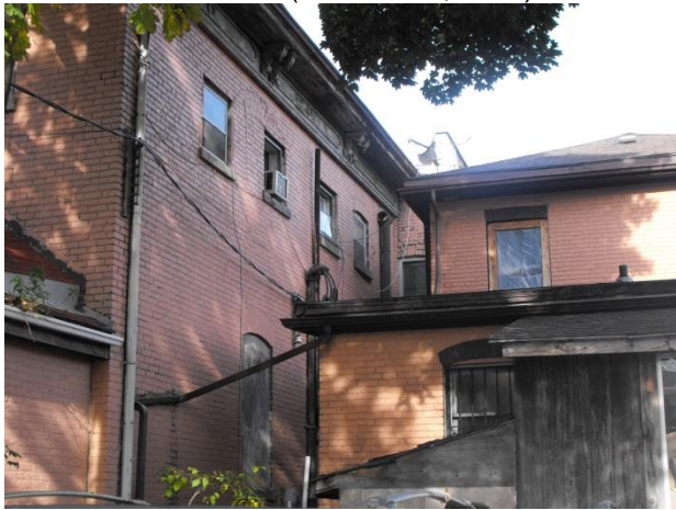
Image 4: East elevation, also showing 451 Dundas Street (adjacent property) (October 24, 2014)
