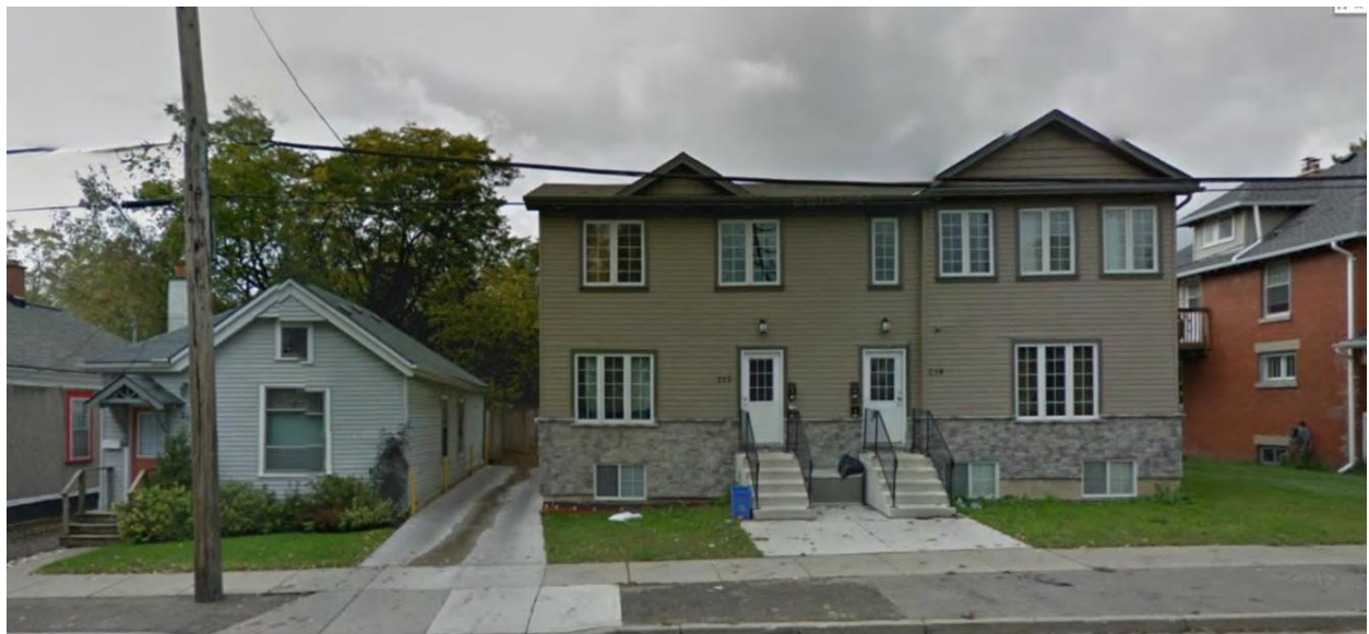
New Building on Wharncliffe Road
