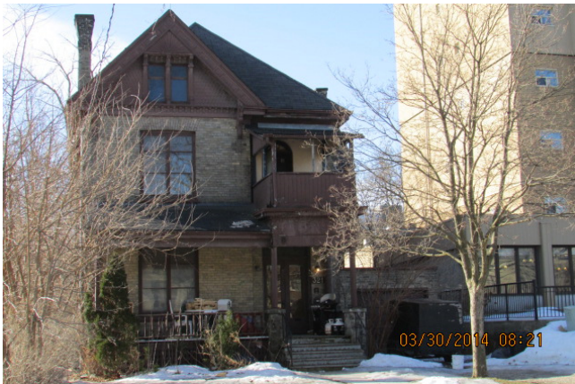
321 Central, to be removed
