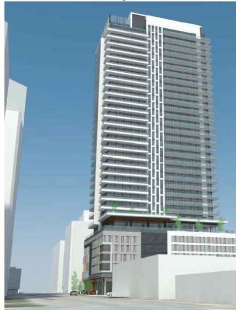
North West Corner of Building
