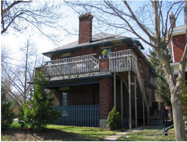
Image 18 - Balcony alteration, 197 Ridout, replication of baluster texture and new stair in unobtrusive location.
