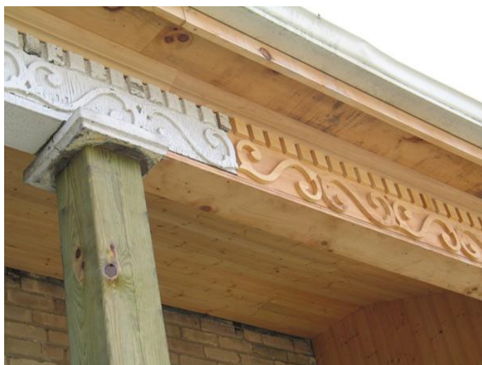
Image 29 - Fascia repair detail, 17 Elmwood
