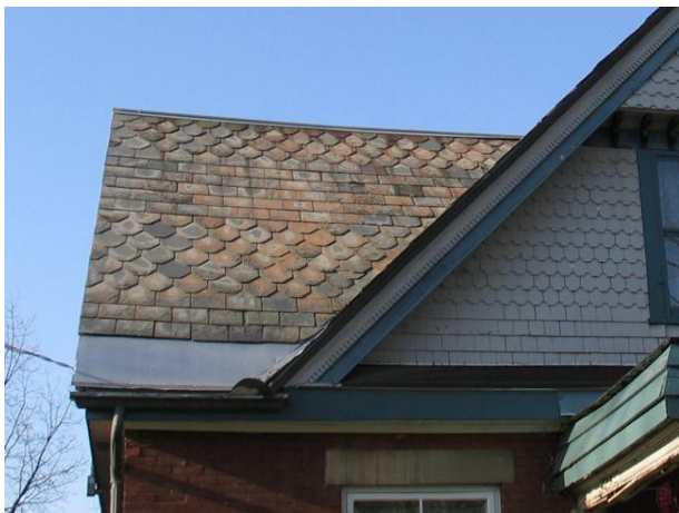
Image 30 - Roofing slates, 88 Duchess
