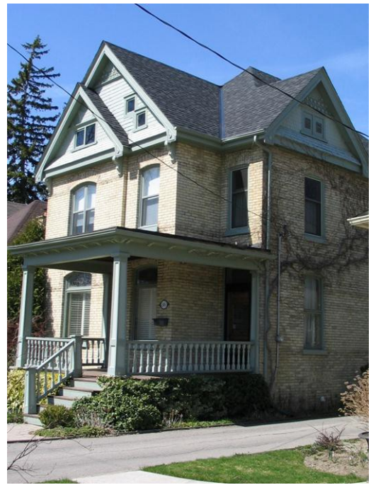
Image 15 - Gabled roof, 86 Elmwood
