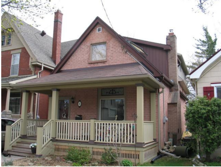
Image 22 - Rebuilt residential, 15 Victor
