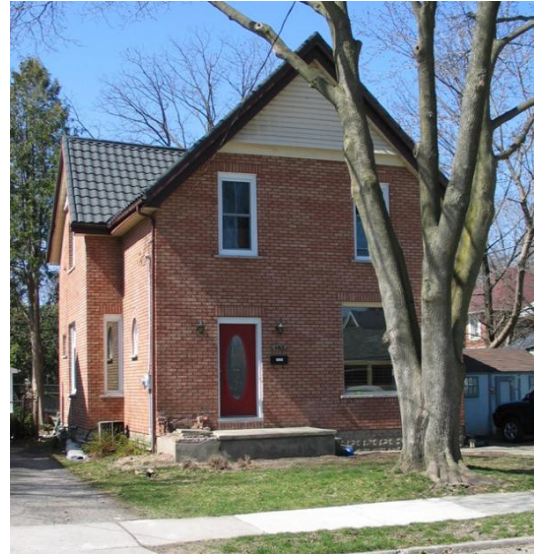
Image 23 - Rebuilt residential, 107 Marley
