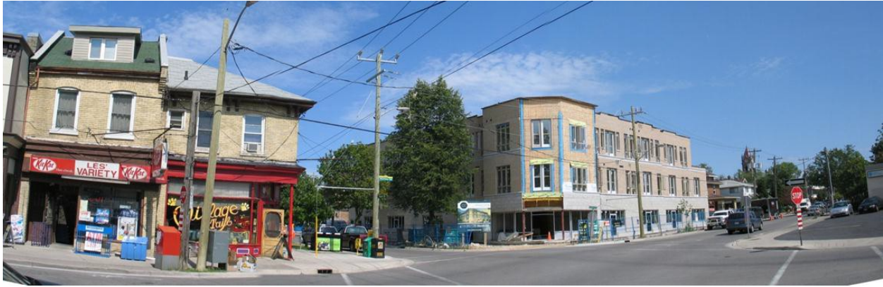
Image 24 - New Commercial Building, 162 Wortley
