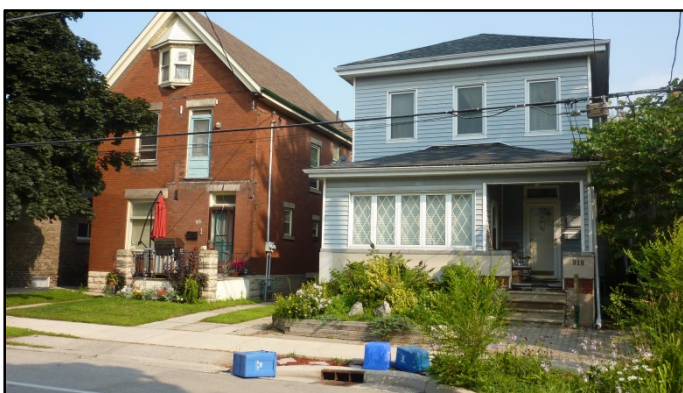
Adjacent properties - east
