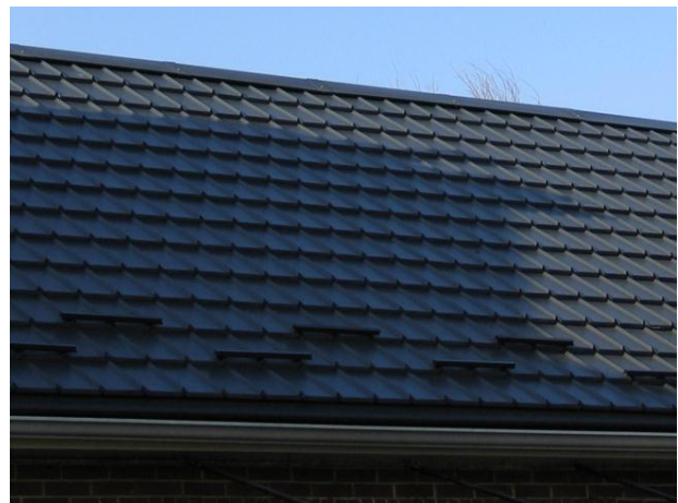
Image 31 - Metal shingles, 96 Duchess
