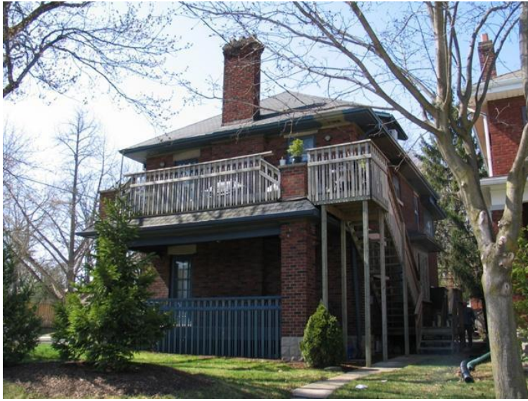
Image 18 - Balcony alteration, 197 Ridout, replication of baluster texture and new stair in unobtrusive location.
