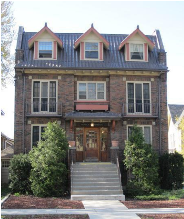
Image 2 - Monica Apartments, 113 Elmwood Avenue, 2010
