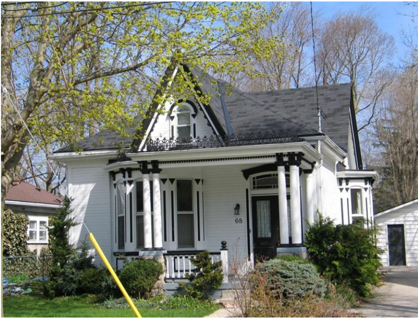
Image 36 - Wood siding, 68 Bruce
