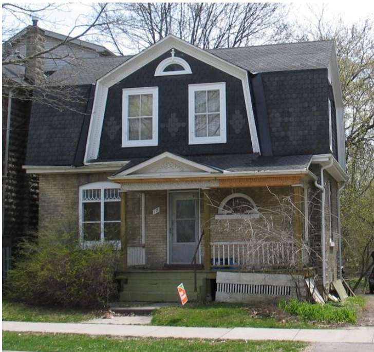
Image 14 - Mansard roof, 17 Elmwood
