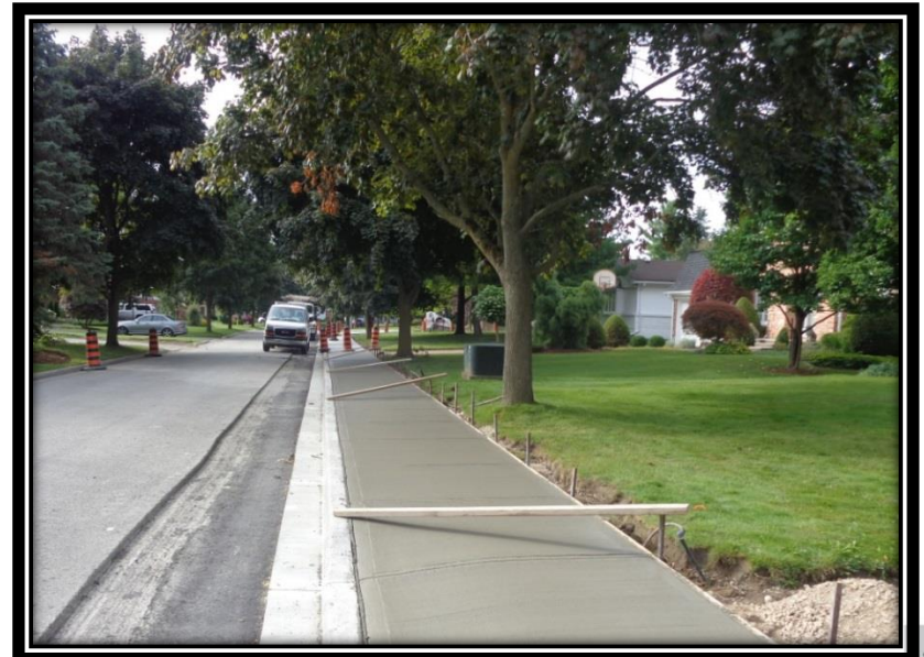
New Curb Faced Side walk Cherokee Road
