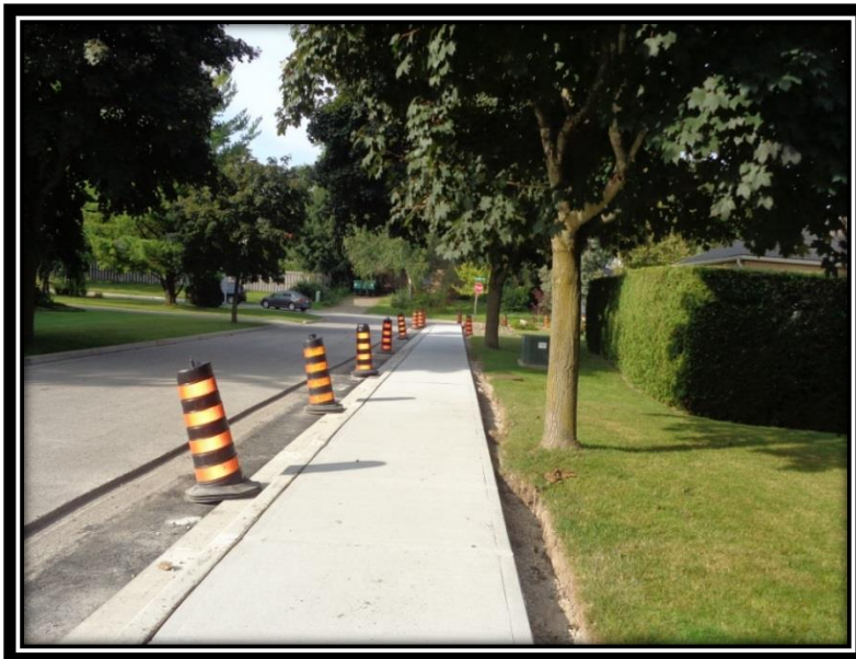
New Curb Faced Sidewalk Cherokee Road
