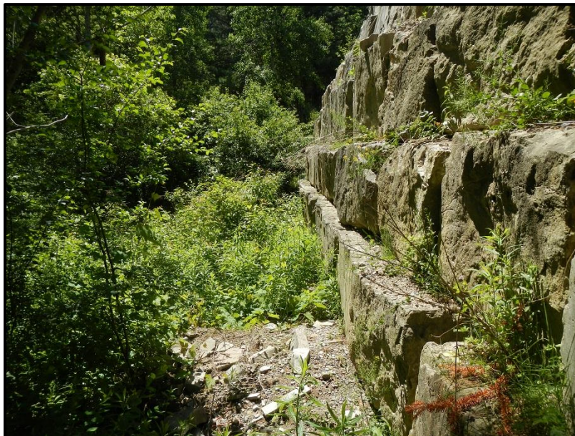
Photo 15. Vegetation along retaining wall at Hunt Club West
