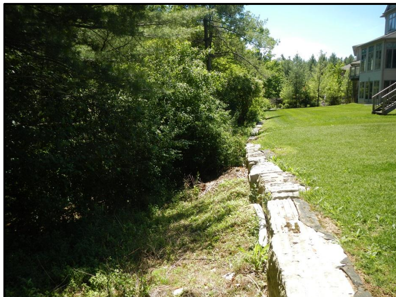
Photo 2. Unfenced lot along segment B at Hunt Club West Riverbend
