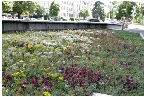
City Hall's green "roof". Photo courtesy of LiveRoof
