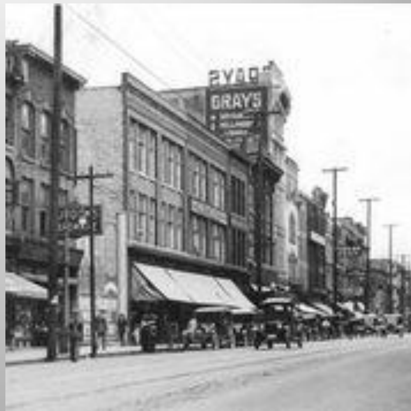
Photograph taken after the 1911 fire – note the empty lot to the west of Kingsmill's
