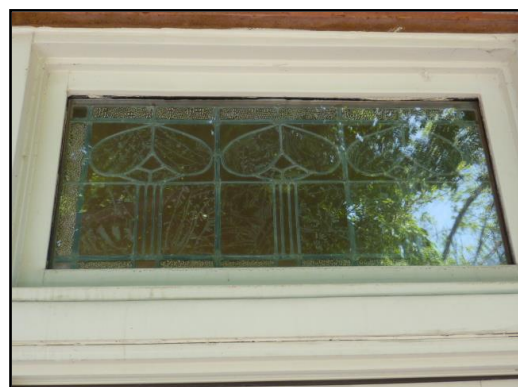
Dining Room transom windows showing relocated leaded glass panels attached inside
