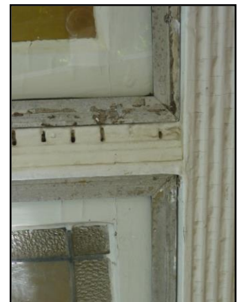
Existing windows - front bay showing aluminium frames
