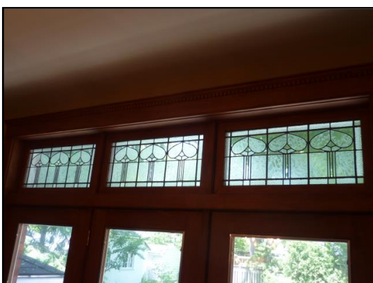
Dining Room transom windows showing relocated leaded glass panels attached inside
