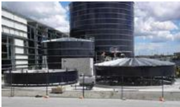
Anaerobic Digestion Facilities Toronto
