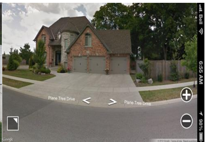
Wide Drive not in compliance to By-laws
