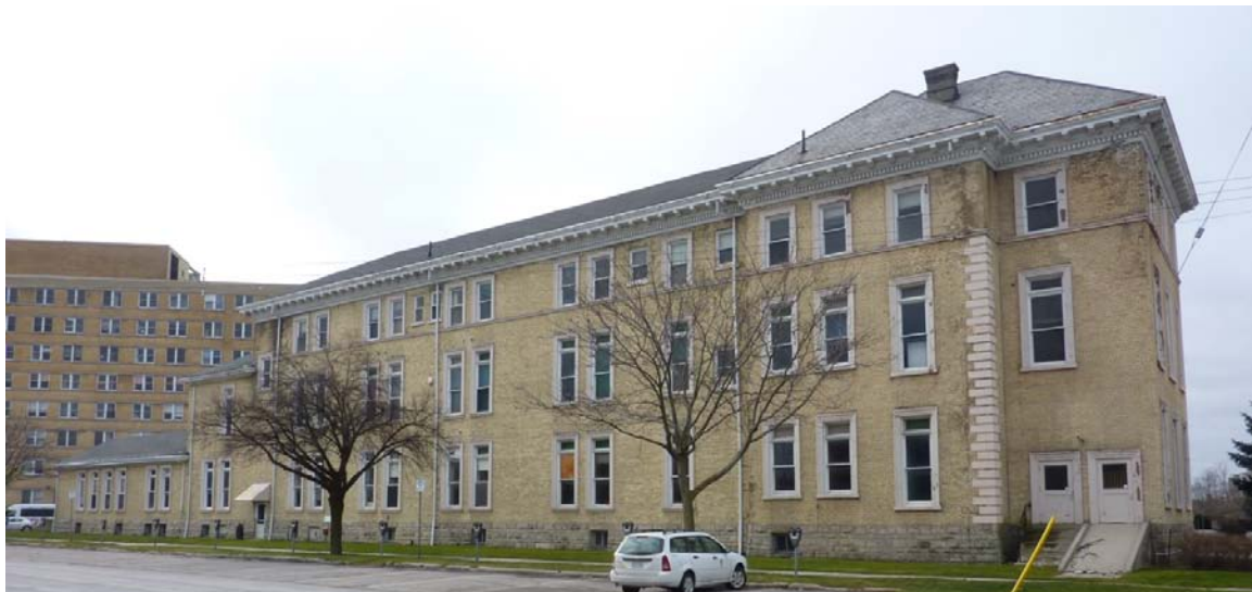
Figure 12: (1) Colborne building, 1899 – Priority 1
