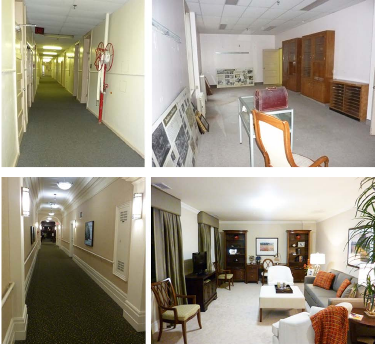
Figure 20: Existing corridor conditions (top left) and interior room conditions (top right) of the Colborne Building. Windermere on the Mount (bottom images) shows how the spaces could be transformed in an adaptive reuse process.
