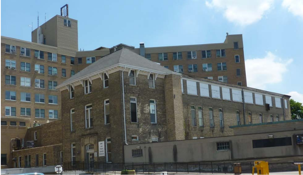
Figure 19: (8) Old Surgical Building (former TB Ward), 1899/1914
