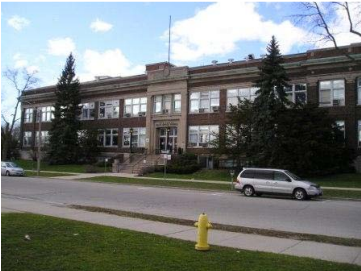
Figure 16: (5) Health Services Building Former Western Medical School, 1921 – Priority 3
