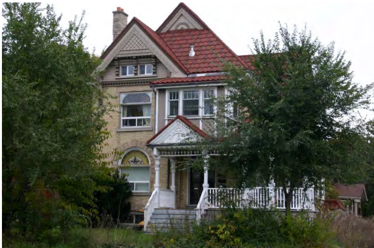
Image 27: 101 Wharncliffe Road North
