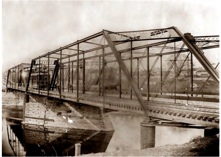
Image 38: The Warren Truss Kensington Bridge (in back) with the railway bridge in front, circa 1909 (Western Archives, University of Western Ontario)
