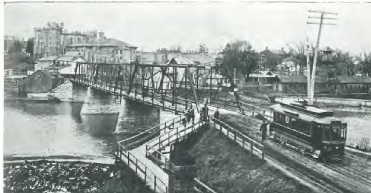
Image19: The West London Streetcar at the west end of the Kensington Bridge, c. 1895
