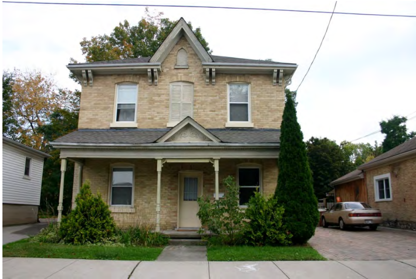
Image 68: 13 Napier Street (1873), London buff brick with Gothic centre gable, paired roof brackets, an asymmetrical entry and front porch
