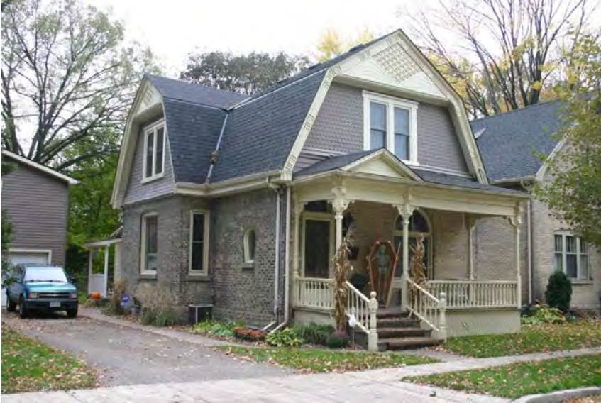
Image 75: 2 Cherry Street, 1909, built for Charles Howey, this 2 storey, hip-roofed house with projecting side bay and gable has the Victorian-style porch which is a contemporary addition (Note the keyhole window)
