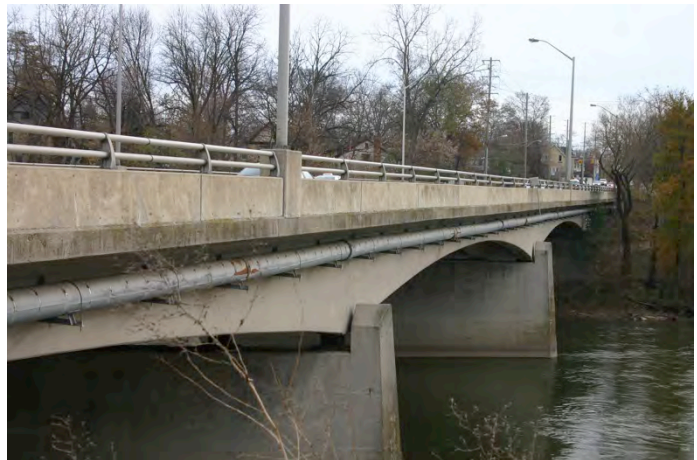
Image 39: Wharncliffe Street Bridge, in 2013
