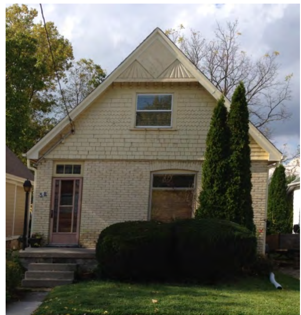
Image 71: 58 Albion Street, built c. 1906 (note "linen-fold" or fan detailing of gable decoration)
