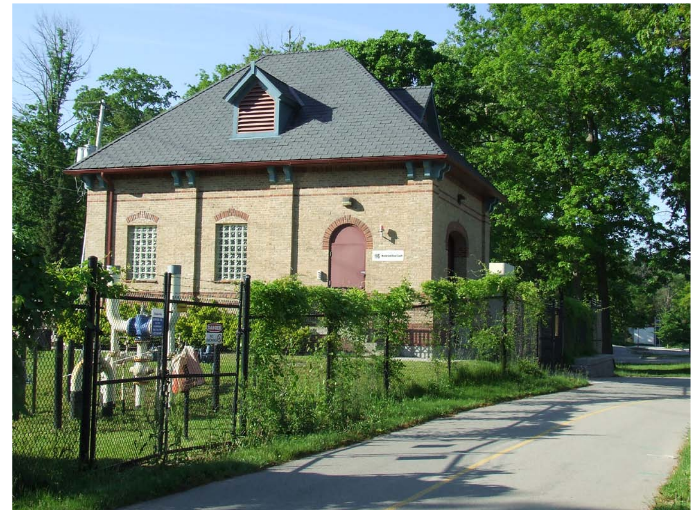
Municipal infrastructure in Springbank Park
