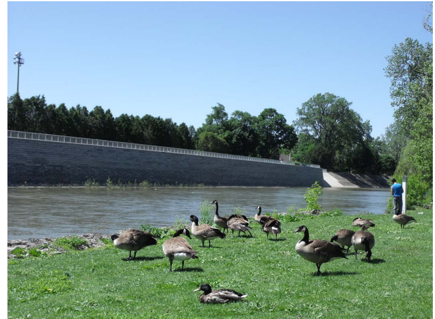
The recently constructed dike located along the west side of the Thames River, opposite Harris Park, won a design award in 2010. The dike protects residents from flooding events.
