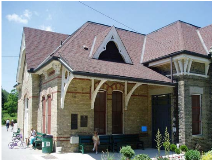
The Pumphouse in Springbank Park is a historic structure on the Thames River remaining from the original London Waterworks and could house a river's edge cafe.
