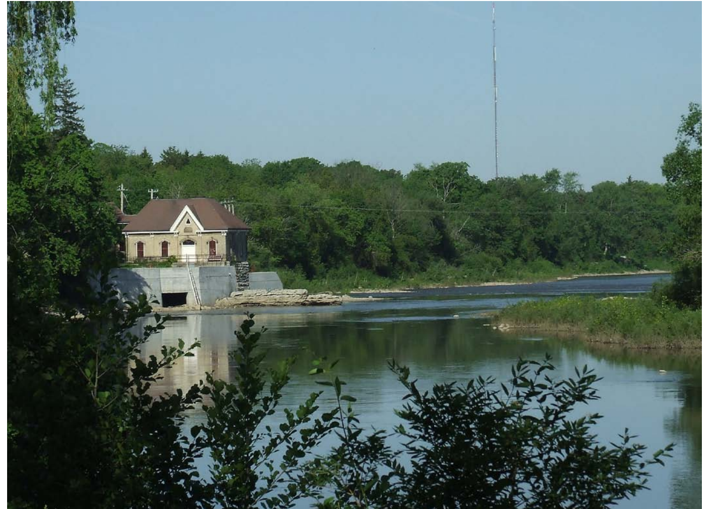
Pumphouse in Springbank Park
