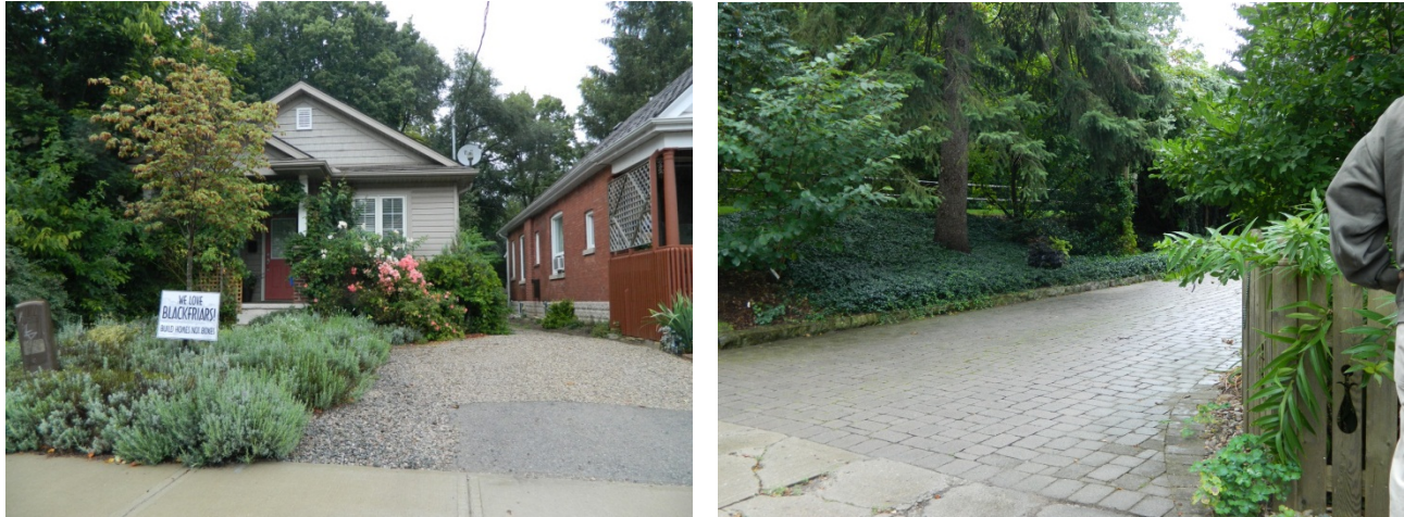
Figure 20: Recommended alternatives to concrete or asphalt include natural colored gravel or decorative pavers.
