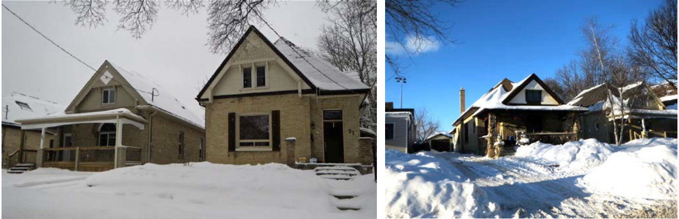
Figure 7: 31 and 33 Charles Street (left) and 35 Charles Street (right). The river stone porch appears to be a later addition.
