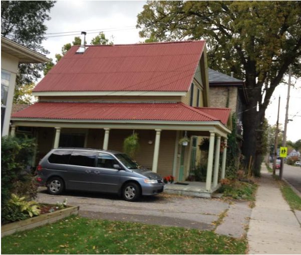
Figure 14: Gable roof with a hipped-roof covered porch
