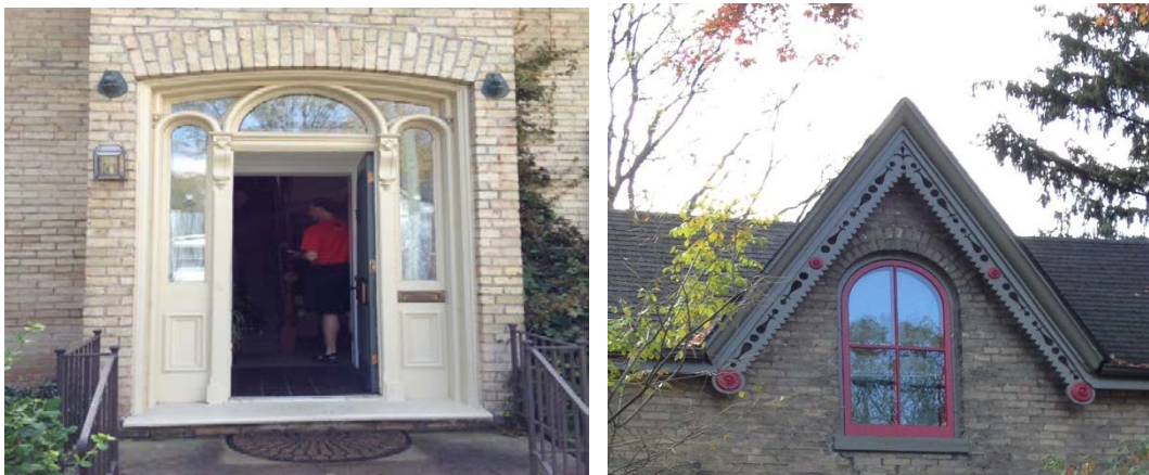
Figure 12: The three-arched, "London" entry door and side lights (left) and 1880s delicate bargeboard and arched dormer window (right).
