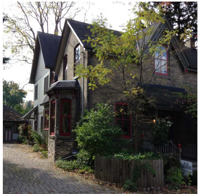
Figure 16: An exterior addition located at the rear of the building and street-facing elevation
