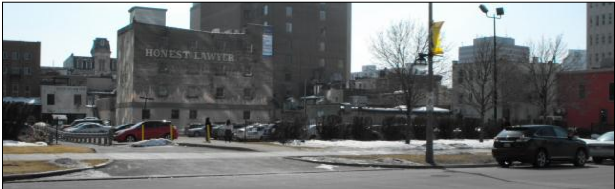
Figure 5 – South facing (front) view of subject lands and exit onto Queens Avenue.
