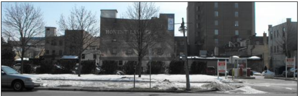
Figure 2 – South facing (front) view of subject lands and entrance from Queens Avenue.
