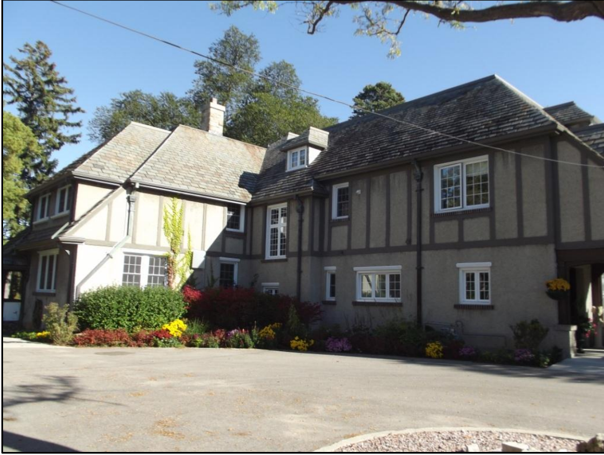
View of Gibbons Lodge from the Southwest
