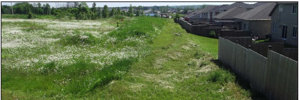
Figure 3 – 2250 Blackwater Road: facing east. Single detached dwellings at significantly lower grade.
