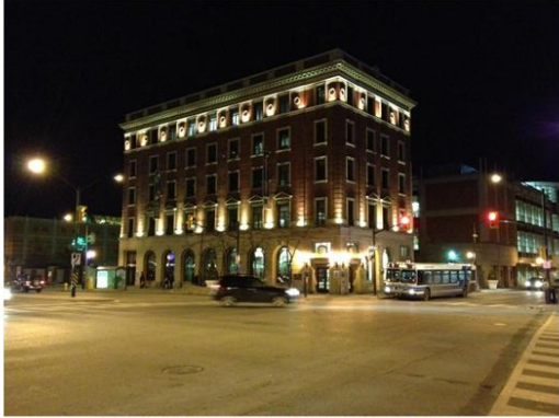
Energy Efficient LED Lights at J. Allen Taylor Building, London, Ontario
