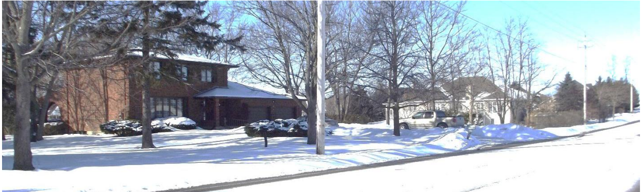
Figure 4 –View of 1055 Wesdel Bourne & 2039 Ashgrove Court, facing northwest on Wesdel Bourne
