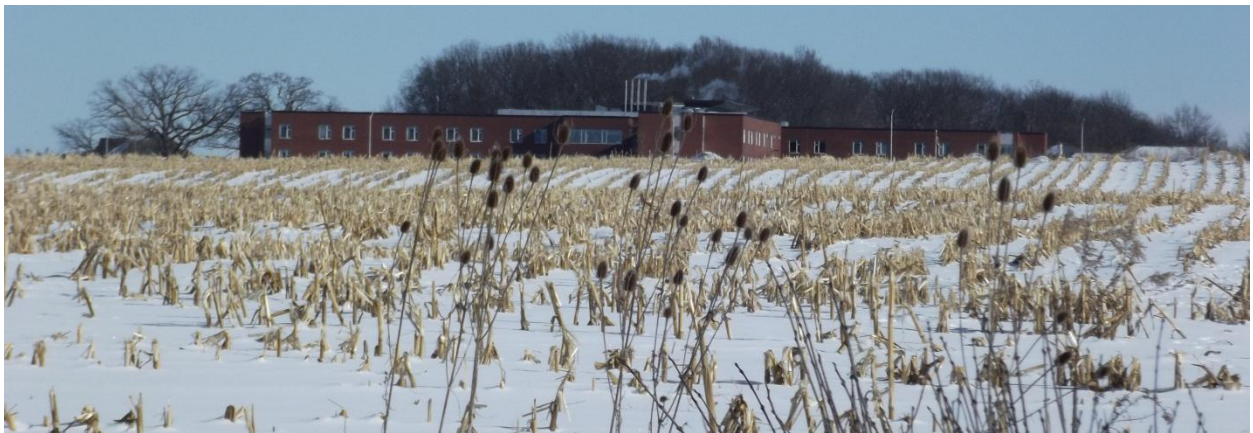
Figure 5 –East facing view of McCormick Nursing Home located at 2022 Kains Road
