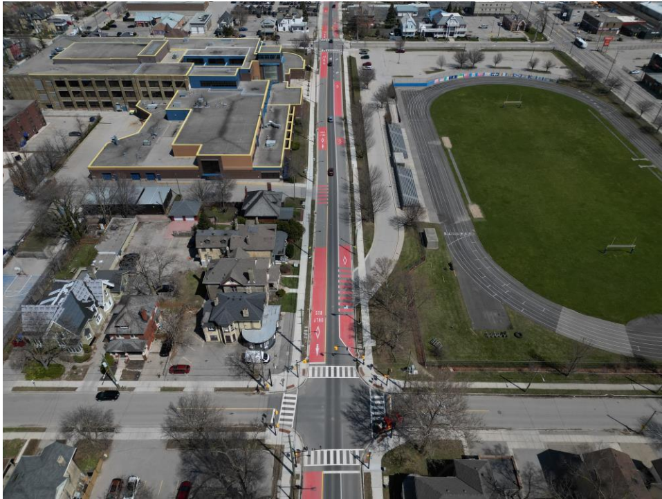
Above: An aerial drone photo of the King Street contraflow bus lanes between Maitland Street and William Street.
