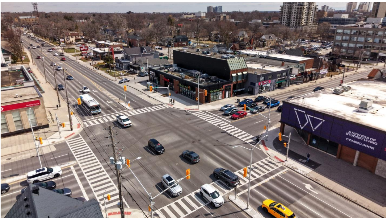
Above: Completed Oxford Street East and Richmond Street intersection improvements
