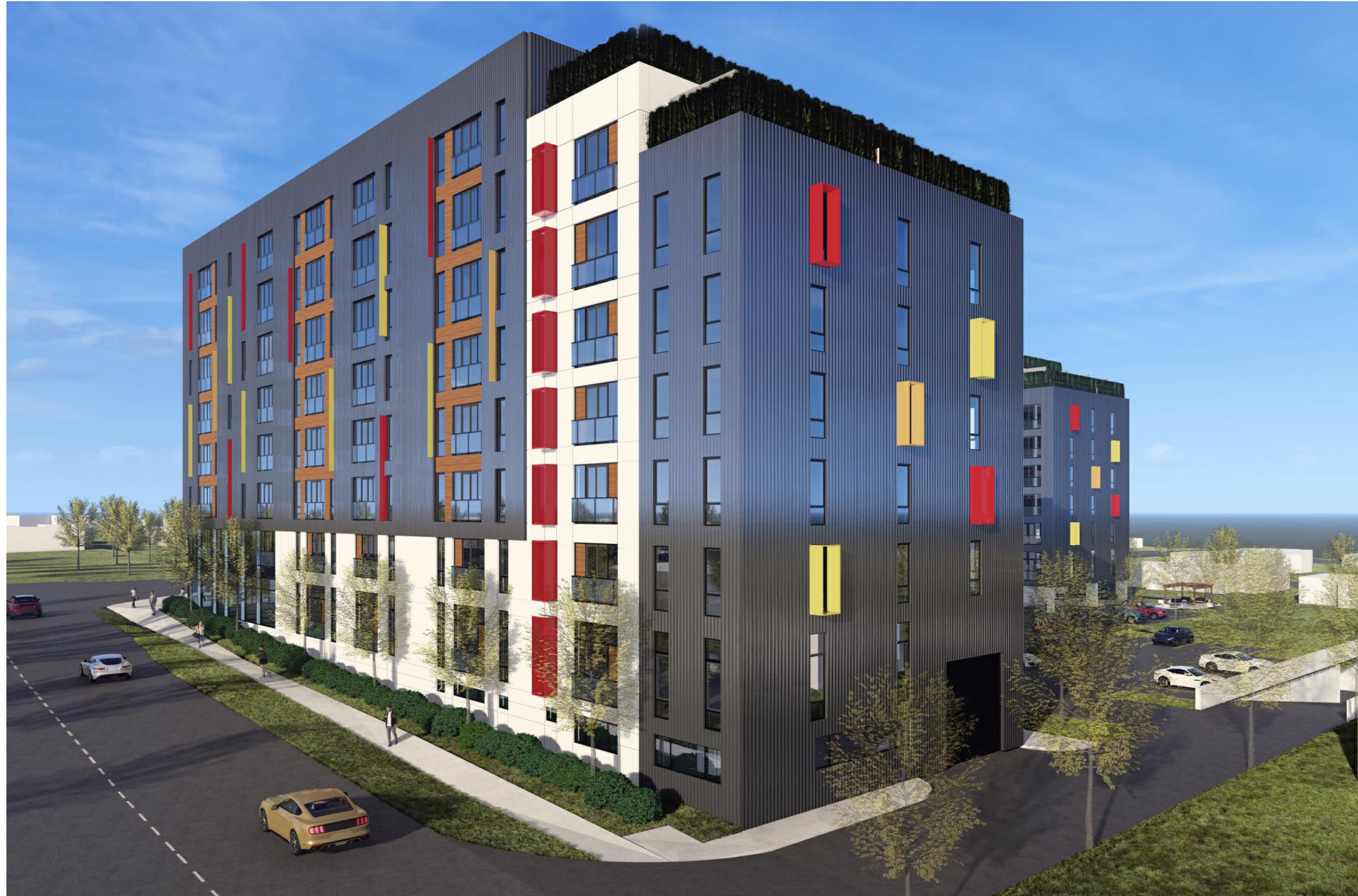
VIEW FROM NEW SITE ACCESS ON GEARY
