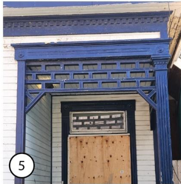
5 Off-set rectangular fretwork with triangular bracing at corners
