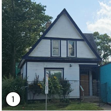
1 One-and-a-half storey, L-shape, cross-gable massing, typical of the Queen Anne style
