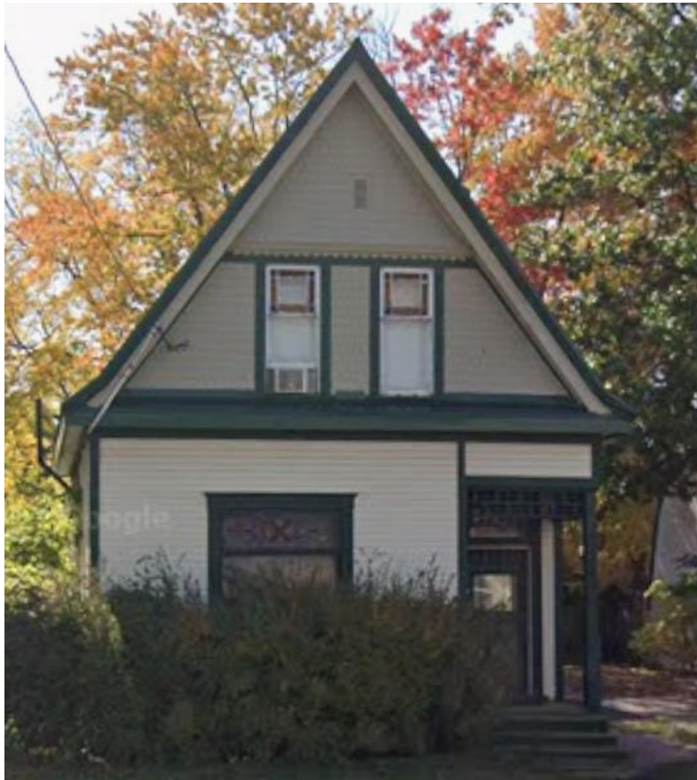
Figure 16 – 377 Hamilton Road, immediately east of the subject lands (Google Street View)
