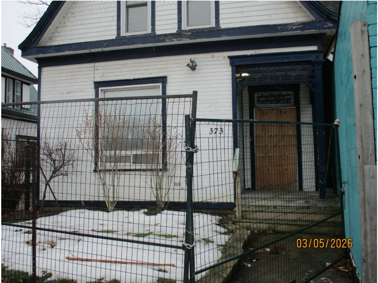
Image 3: Photograph showing the ground storey and entry to the building at 373 Hamilton Road.
