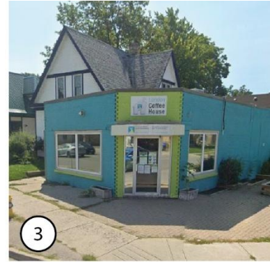
3 Chamfered corner facing the intersection of Hamilton Road and Redan Street
