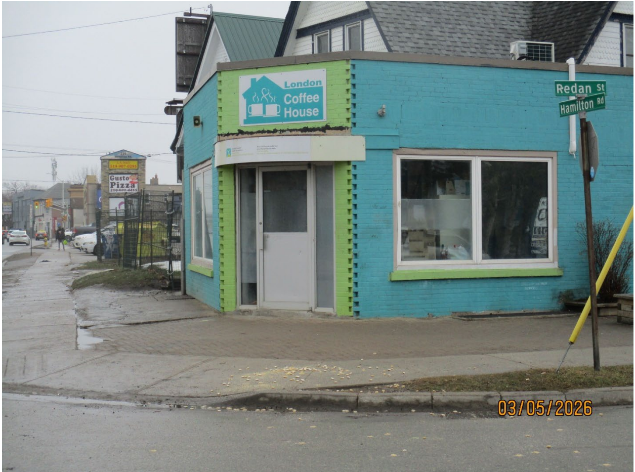
Image 5: Photograph showing the corner entry to the building at 371 Hamilton Road, including sawtooth brick corner detailing.
