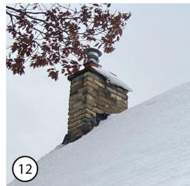
12 Buff brick chimney at the rear, simple brick detailing
