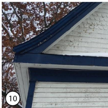
10 Simple wood trim at each corner of the building, painted navy
