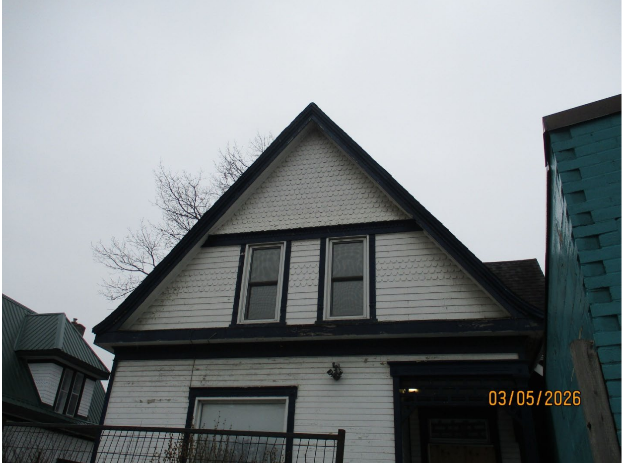
Image 4: Photograph showing the gable detailing on the building at 373 Hamilton Road.
