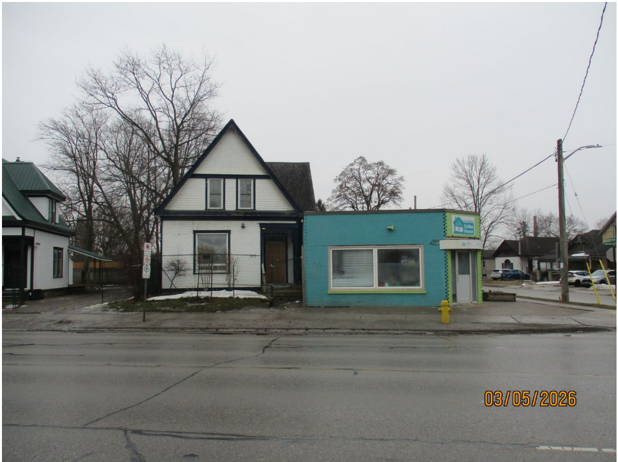
Image 1: Photograph showing the buildings on the heritage listed property at 371-373 Hamilton Road. The residential form building on the left is addressed as 373 Hamilton Road and the commercial form building on the right is addressed as 371 Hamilton Road.
