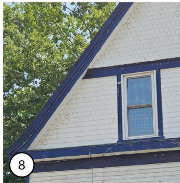
8 Alternating courses of horizontal drop siding and hexagonal wood shingles
