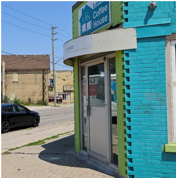
Figures 11-12 – Pigeonhole brick detail at the corner (left), running bond and soldier course patterning (right)
