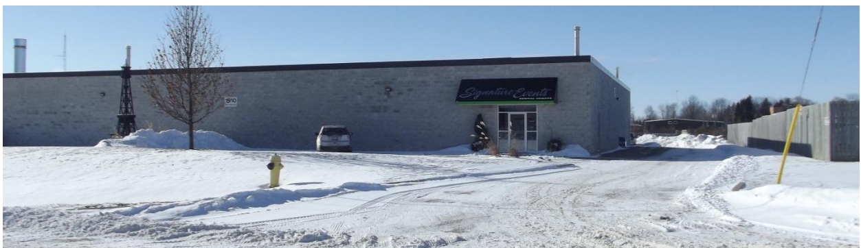
Figure 4 – West facing view of 1910 Blue Heron Drive from road.
