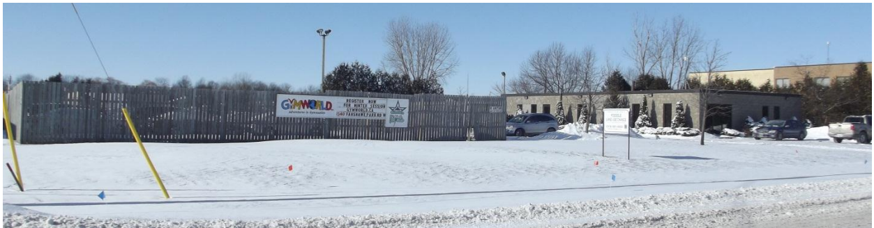
Figure 3 – West facing view of 1920 & 1930 Blue Heron Drive from road.
