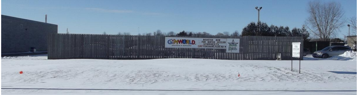
Figure 1 – West facing view of 1920 Blue Heron Drive from road
