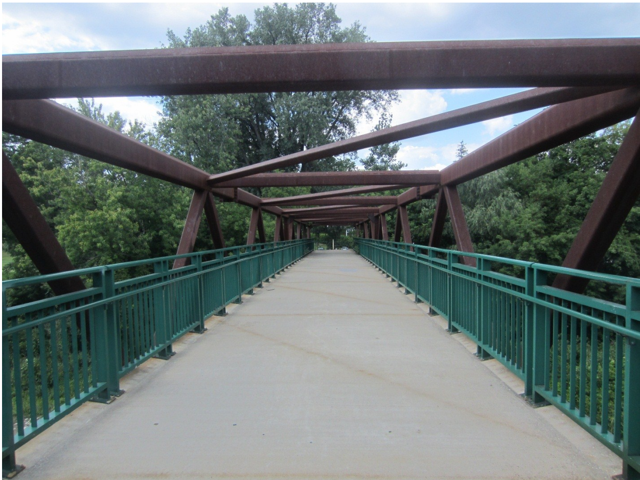
Picture 38 Springbank Pedestrian Bridge
