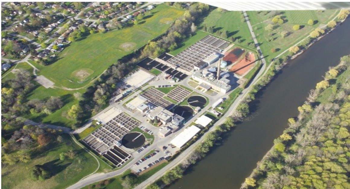
Picture 30 Greenway Wastewater Treatment Plant
