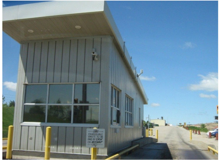
Picture 51 W12A Landfill Entrance
