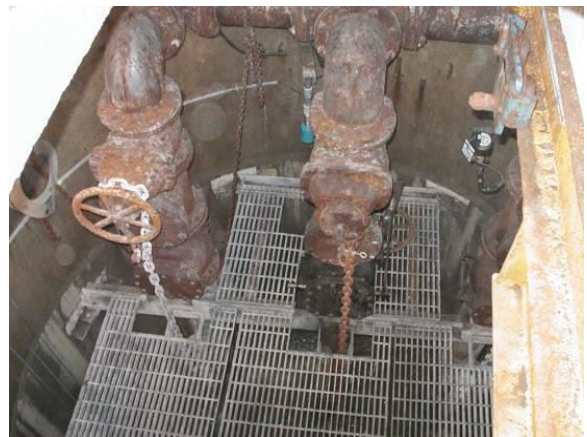
Picture 29 Wet Well at Sunninghill Pumping Station – Scheduled for Decommissioning in 2013
