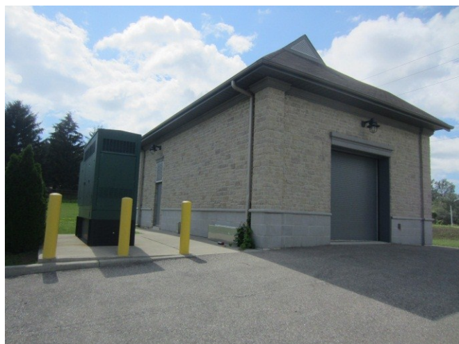
Picture 23 Sunningdale Water Pumping Station
