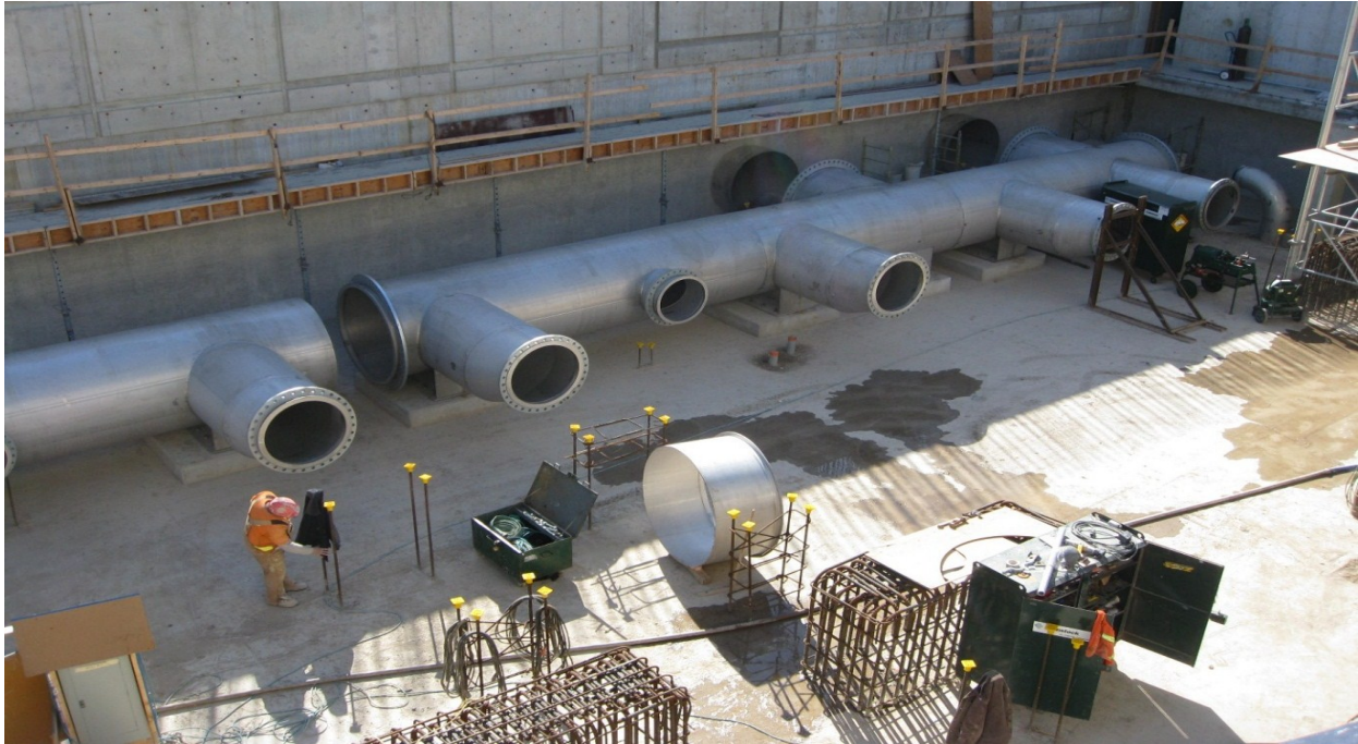
Picture 19 Southeast Reservoir Construction
