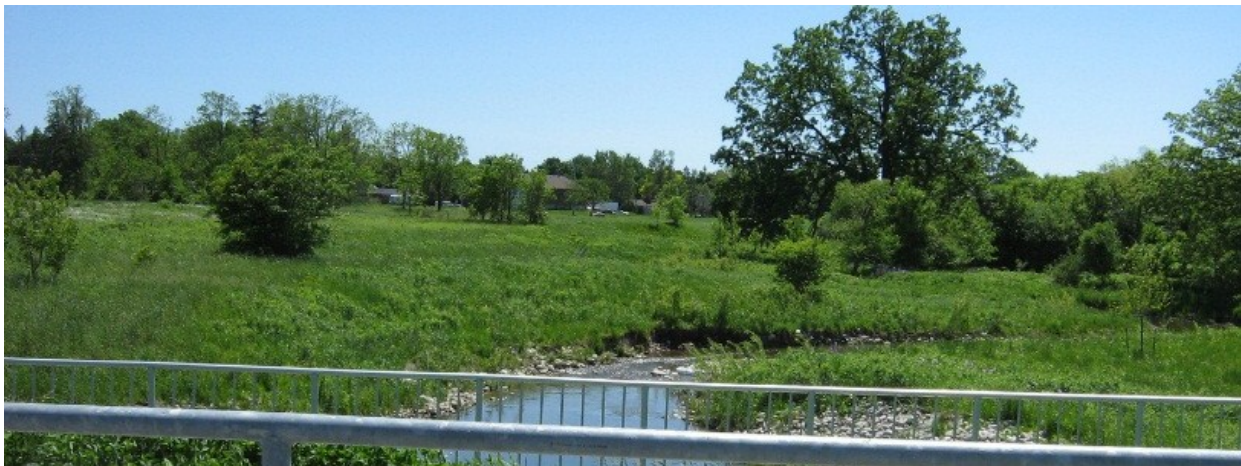
Picture 86 Stoney Creek Flood Control facility
