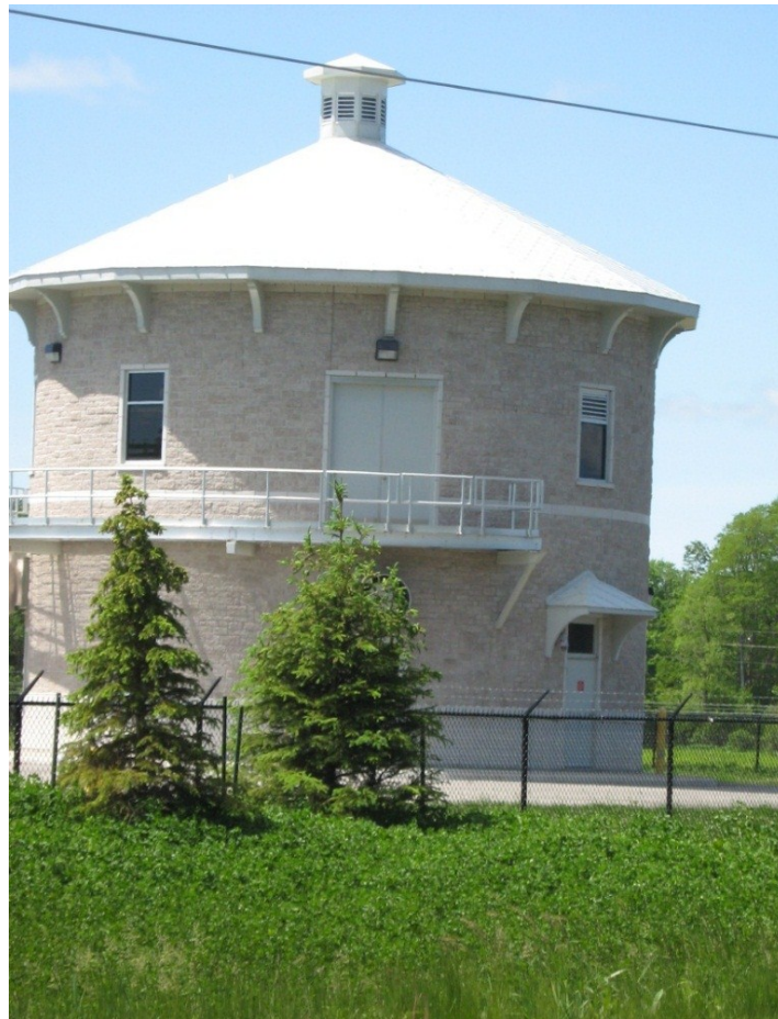
Picture 17 - Dingman Road Pump Station
