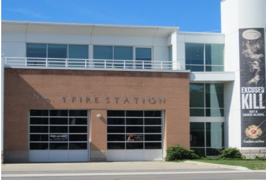
Picture 65 Fire Station No. 1
