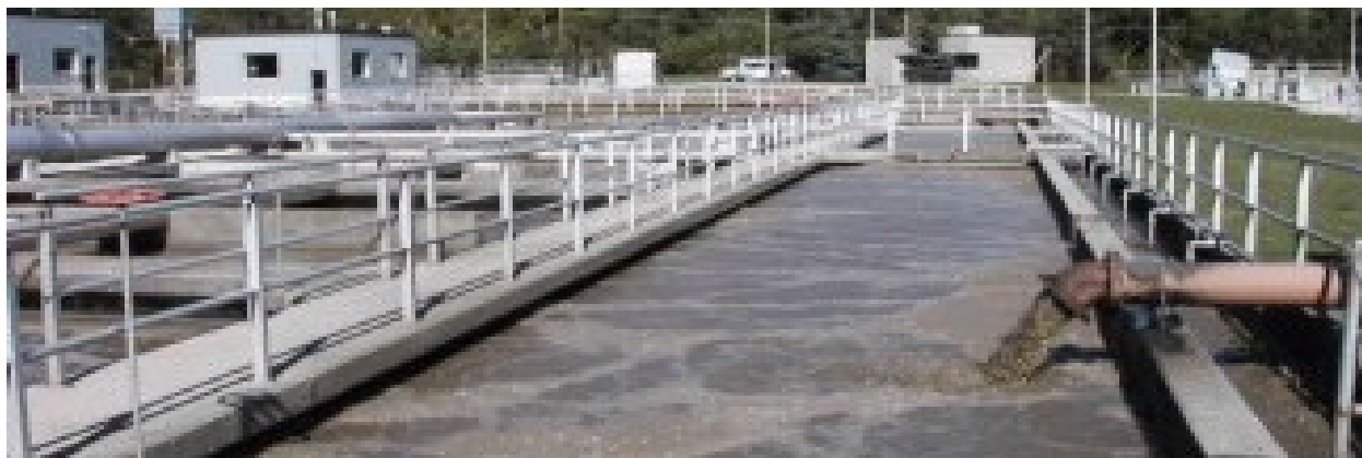
Picture 27 Vauxhall Wastewater Treatment Plant
