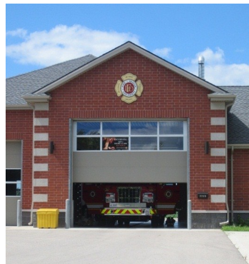
Picture 68 Fire Station No. 14
