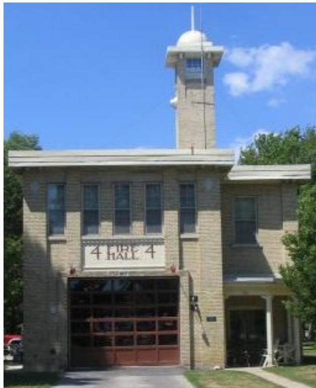
Picture 66 Fire Station No. 4
