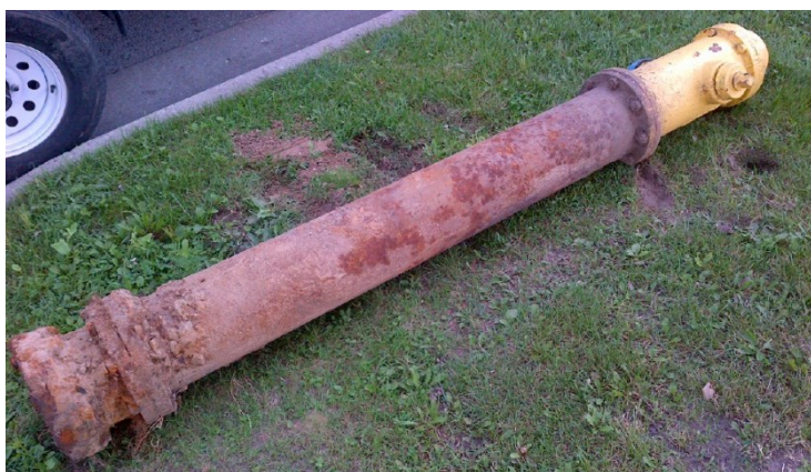
Picture 21 Fire Hydrant Removal
