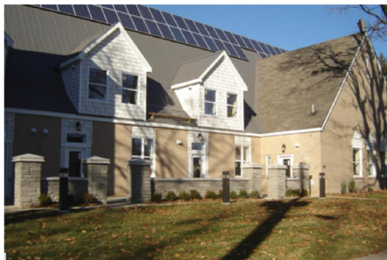
former church on Grosvenor Avenue converted to affordable housing (London, Ontario)
