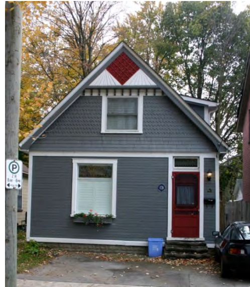
Image 71: 12 Cherry Street, built in 1912 for Joseph Benson (Note "linen-fold" or fan detailing of gable decoration)
