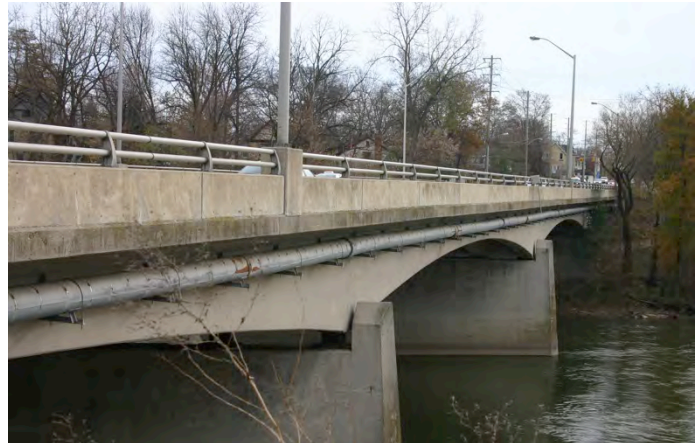
Image 40: Wharncliffe Street Bridge, in 2013
