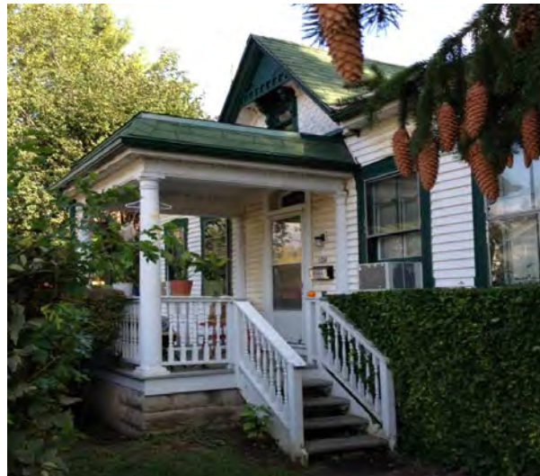
Image 64: 123 Wilson Avenue, 3 bay, Georgian Cottage with Gothic Revival centre gable and later Queen Anne porch built in 1879/1880, probably by the owner, Abraham Bending, who was a mason.
