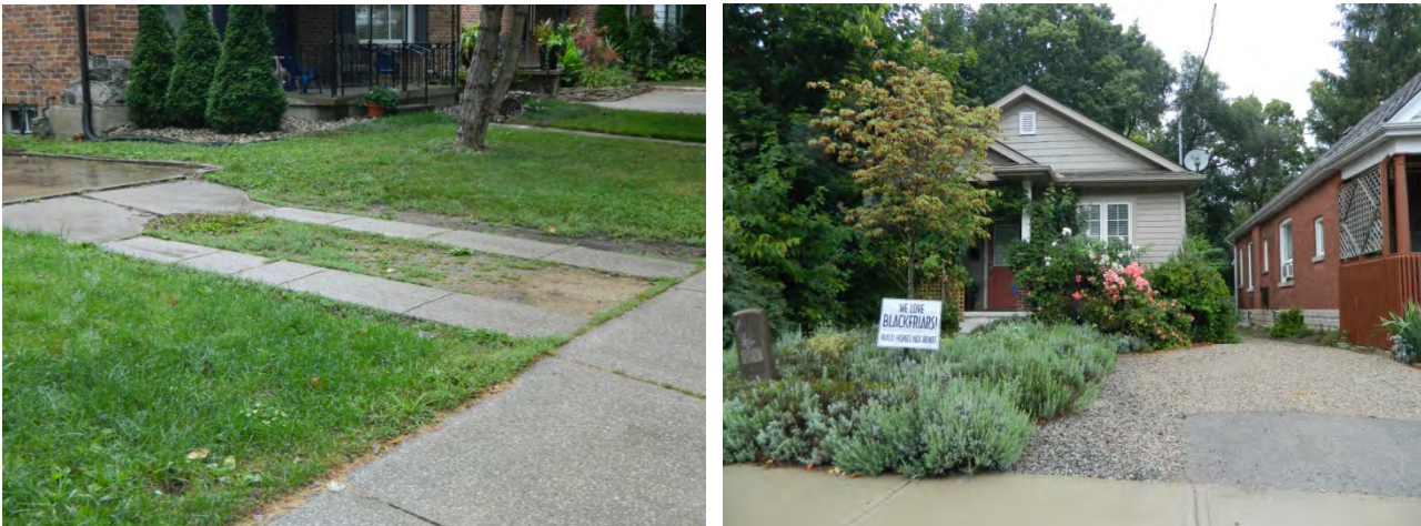
Image 90: A two-track driveway eliminates impervious pavement and enhances greenness of streetscape, and gravel is used as an alternative to asphalt or concrete, creating softer, more natural aesthetic
