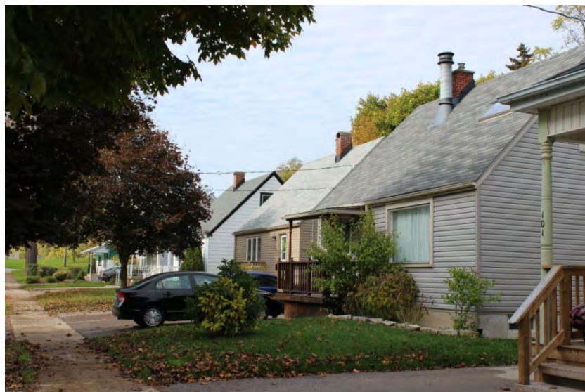
Image 79: A row of Victory Houses shows uniformity in massing, alignment, and architectural style that creates a strong pattern throughout most of Character Area 4, Cavendish Crescent
