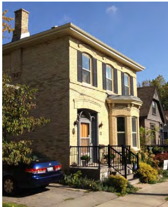
Image 70: 11 Leslie Street, 2 storey, 3 bay, side-hall plan house with Italianate detailing, Likely, and unexpectedly, built as late as c. 1890, after it was purchased by bricklayer Samuel Moore. The Italianate London Doorway, (Note vernacular entry with arched sidelights and transom) the segmental arches over the doors and windows, and the bracketed bay window are all consistent with the Italianate style
