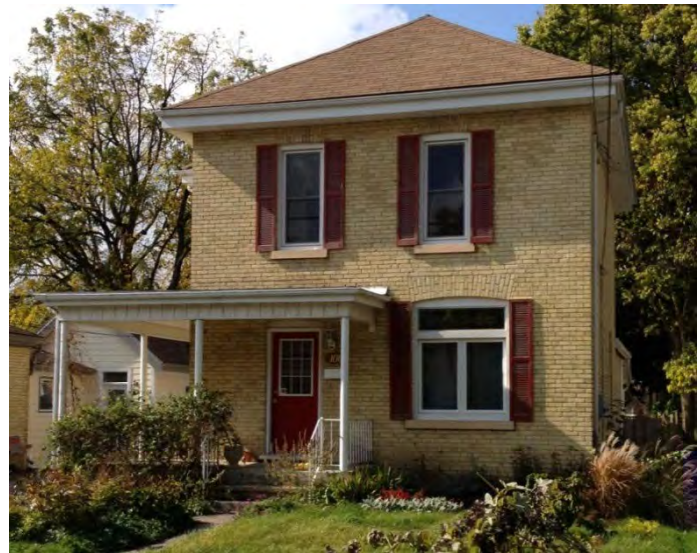
Image 75: 100 Wilson Avenue, built c. 1914
