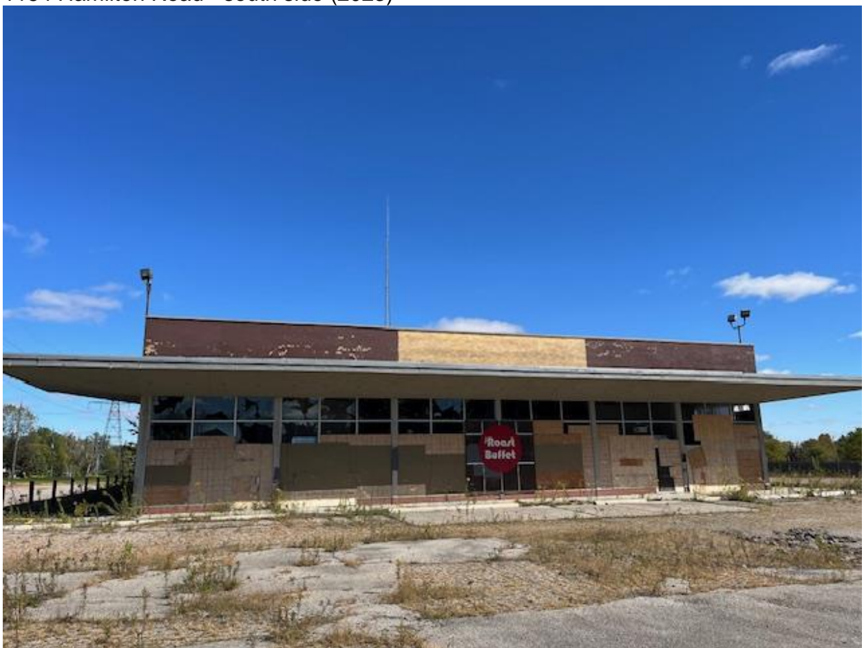
1154 Hamilton Road – façade (2024)
