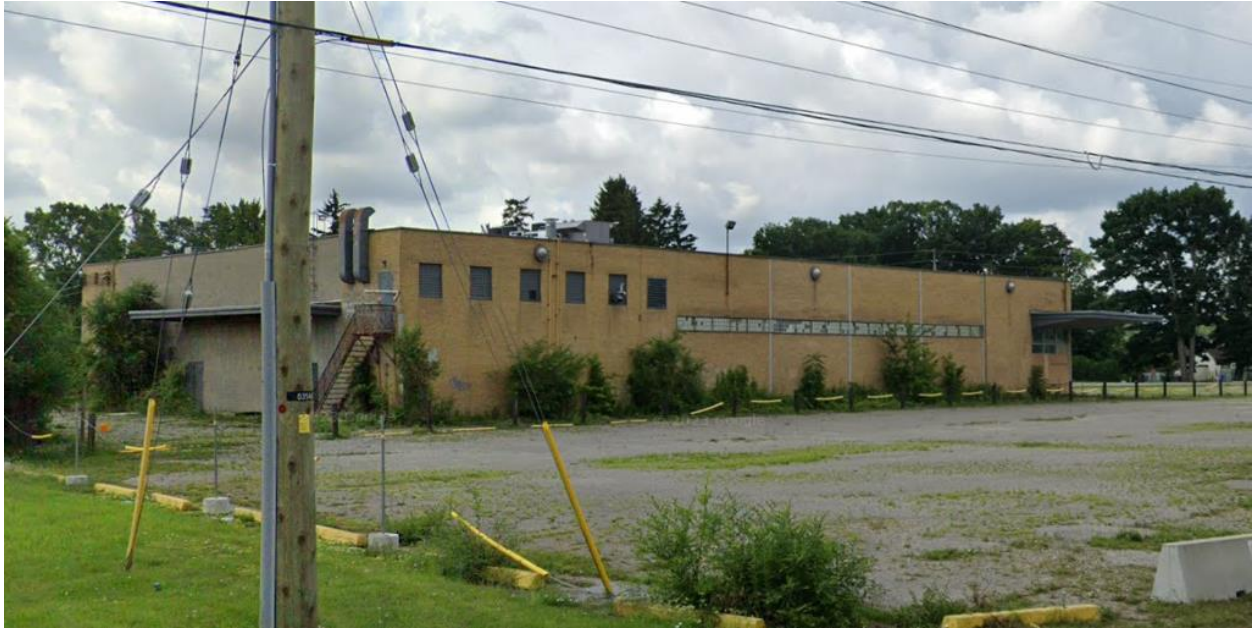
1154 Hamilton Road (north side, 2023)
