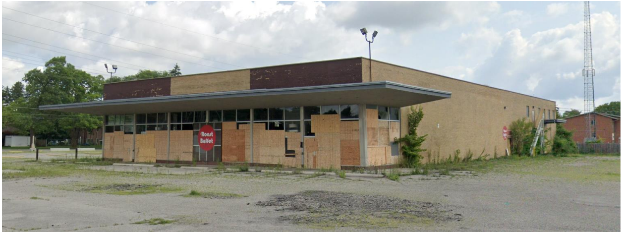
1154 Hamilton Road - south side (2023)
