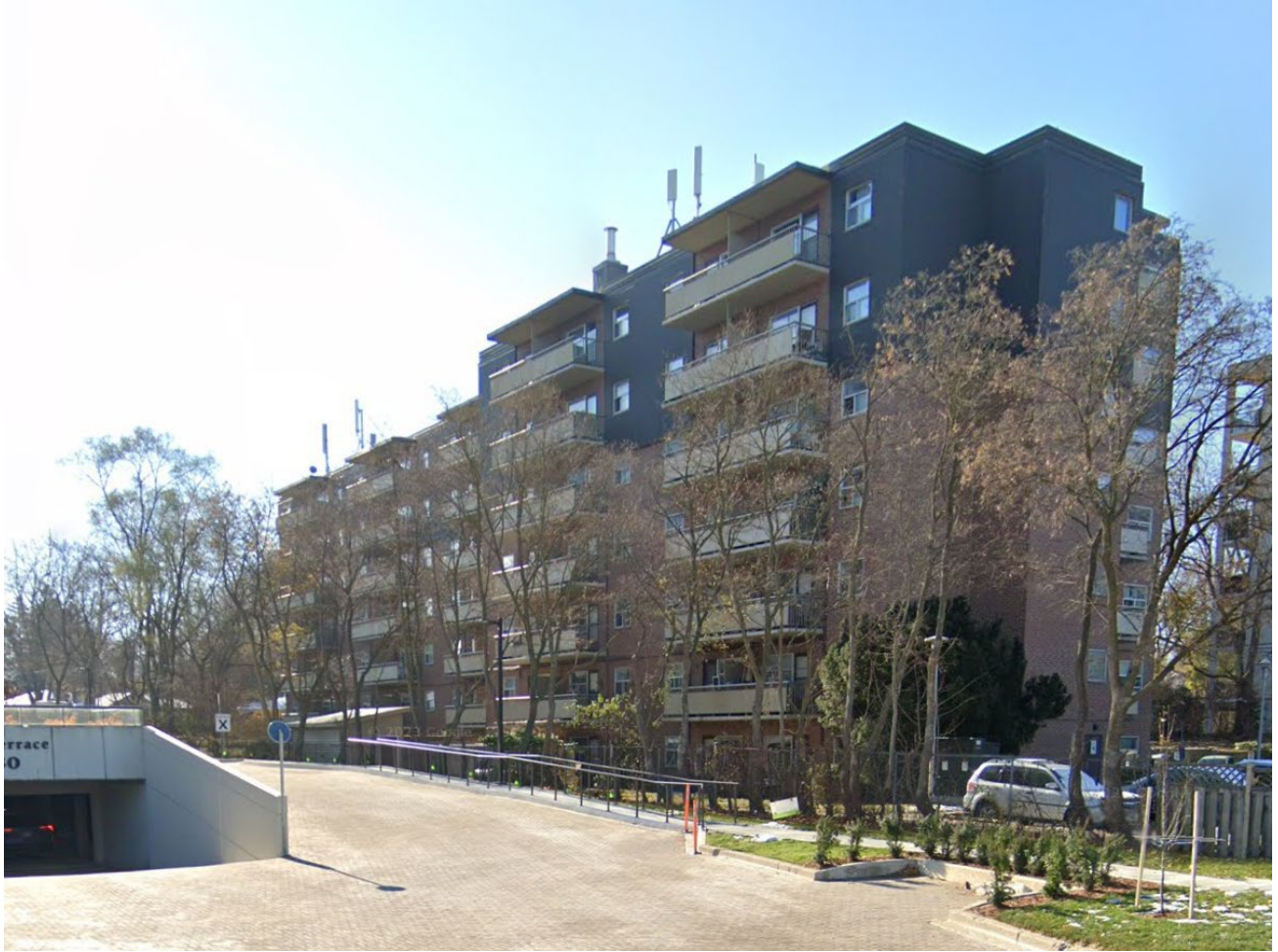
570 Gainsborough Road 7 Storeys Located on Civic Boulevard Adjacent to two storey town homes
