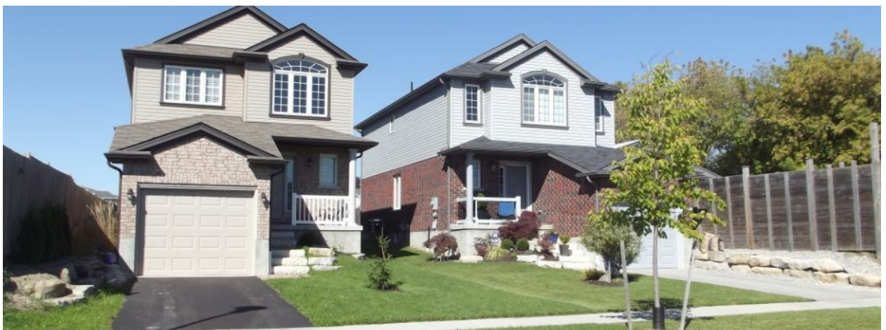
Figure 4 – 1224 and 1226 Savannah Drive
