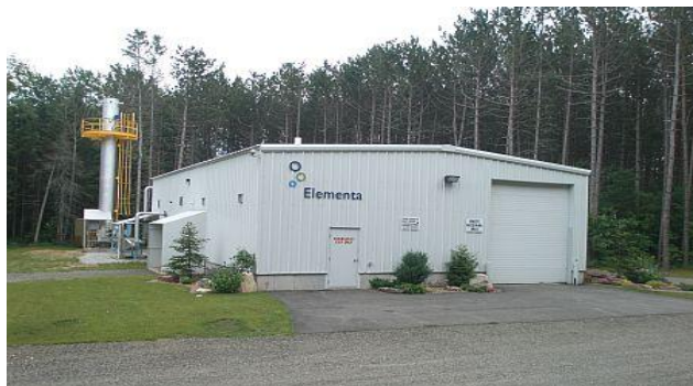
Gasification Pilot Project (Elementa) Sault St. Marie
