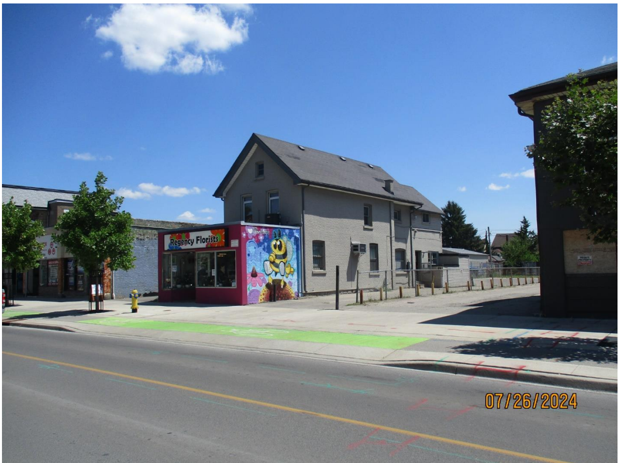
Image 2: Photograph showing the west façade of the building on the property at 773 Dundas Street.
