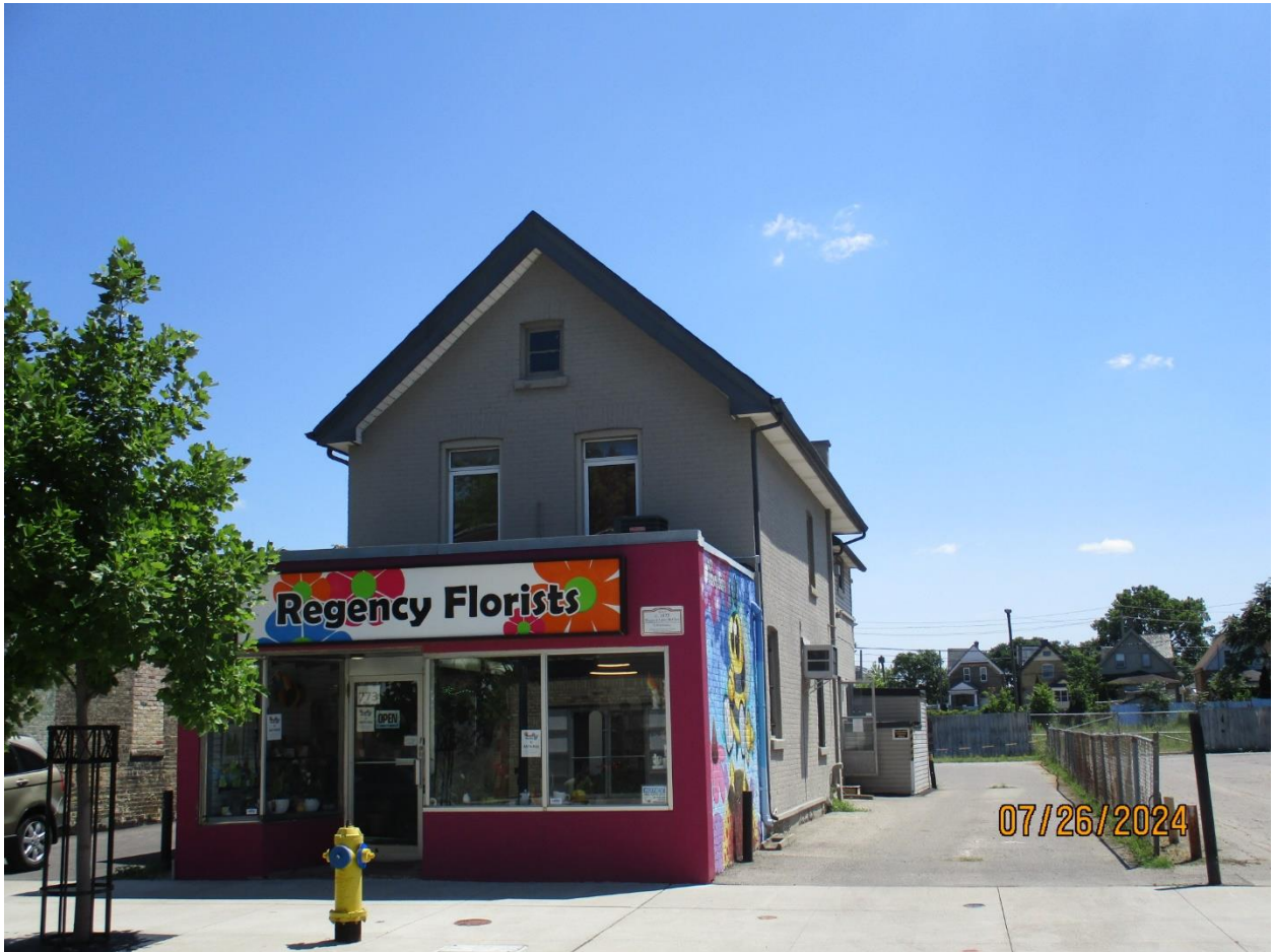
Image 1: Photograph showing the front (north) façade of the building on the property at 773 Dundas Street.
