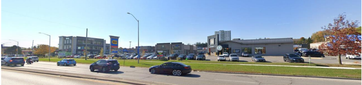
Figure 3 - Streetview of Subject Lands looking west (Google Streetview)
