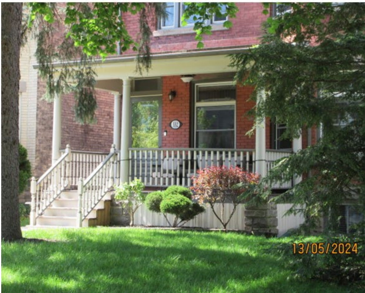
Figure 2: Photographs of the house at 332 St James Street, Bishop Hellmuth Heritage Conservation District. Top, showing the porch prior to 2010. Bottom, showing the porch following its replacement with a porch approved in a Heritage Alteration Permit application in 2010 (bottom photograph taken May 13, 2024).
