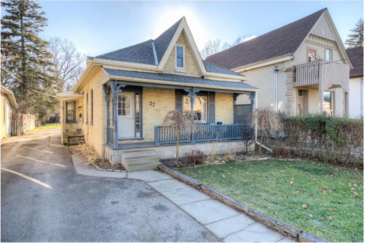
Image 6: Photograph of the house at 27 Bruce Street showing the previous porch prior removal without Heritage Alteration Permit or Building Permit approval. The porch posts and railings consisted of wood materials. The decorative brackets were also removed.
