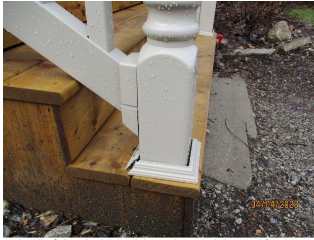
Image 8: Photograph showing detail of the vinyl (plastic) porch materials used for the replacement of the porch at 27 Bruce Street within the Wortley Village-Old South Heritage Conservation District.
