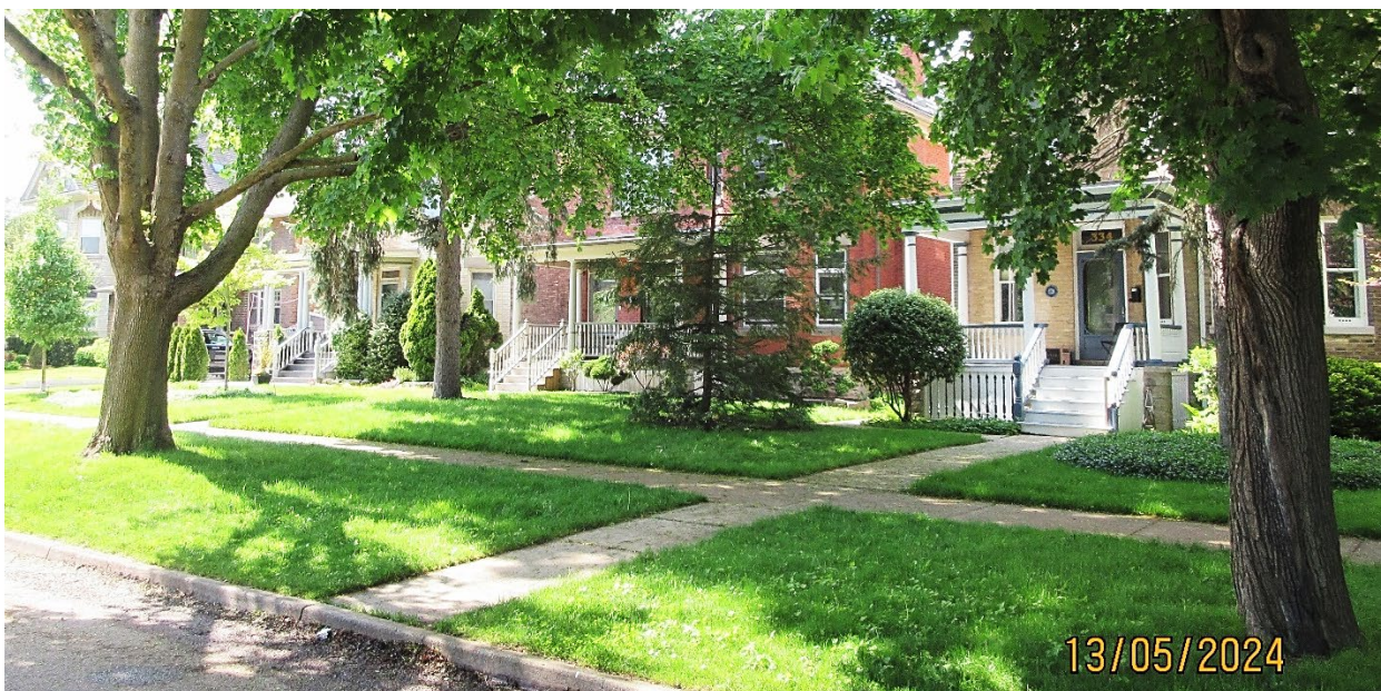
Image 2: Photograph showing the similarly designed houses at 330 St James Street, 332 St James Street, and 334 St James Street (taken May 13, 2024).
