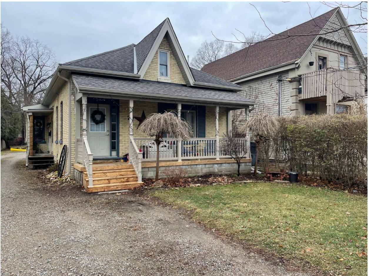
Image 7: Photograph of the house at 27 Bruce Street showing the porch with vinyl-clad (plastic) posts and vinyl railings, with pressure-treated decking.
