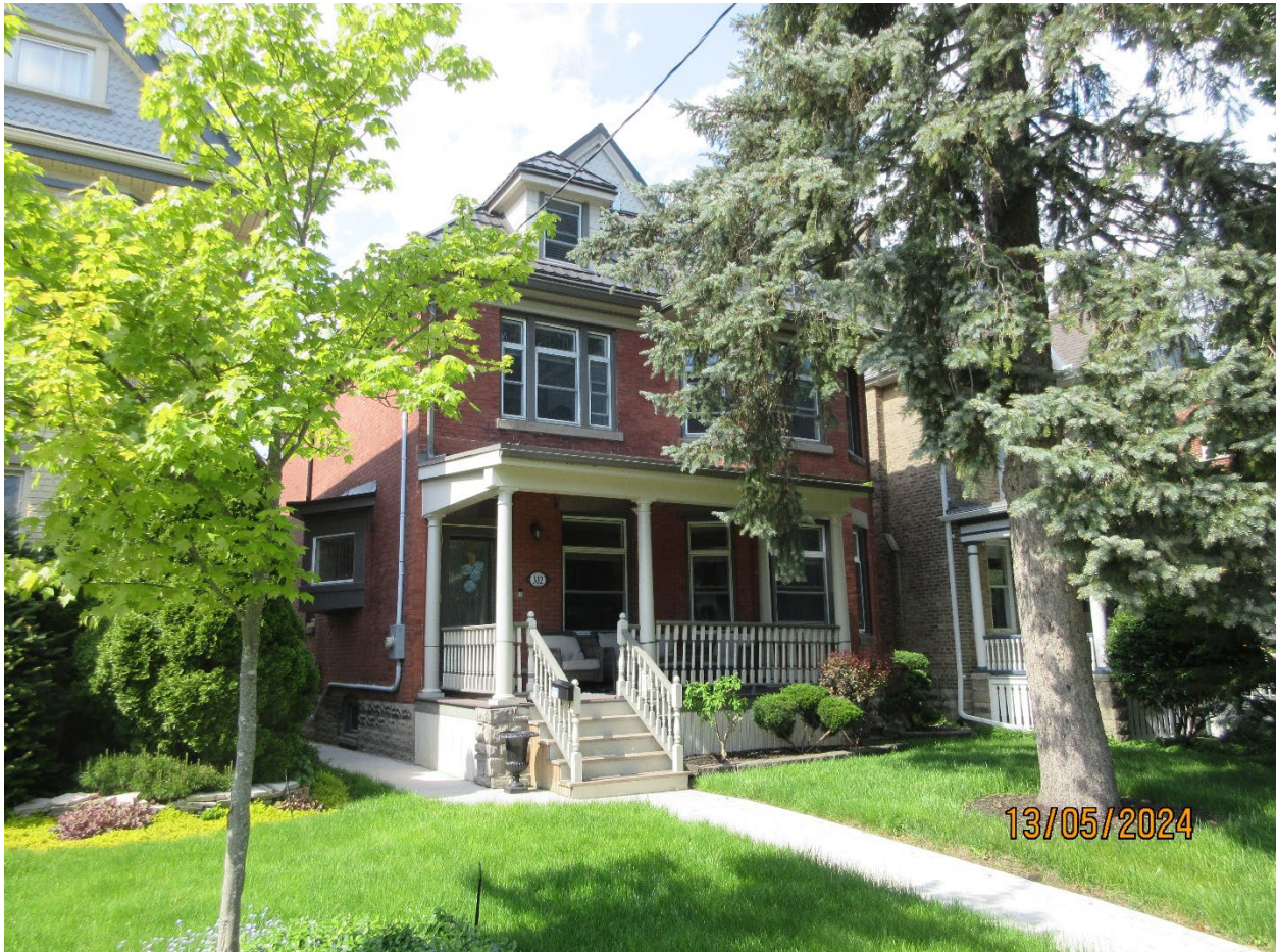
Image 1: Photograph showing the house on the property at 332 St James Street with existing wood porch on the front of the house. The porch railing and newel posts consist of wood materials with a painted finish (taken May 13, 2024).
