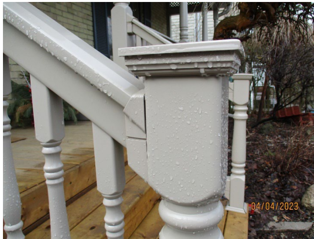
Image 9: Photograph showing detail of the vinyl (plastic) porch materials used for the replacement of the porch at 27 Bruce Street within the Wortley Village-Old South Heritage Conservation District.
