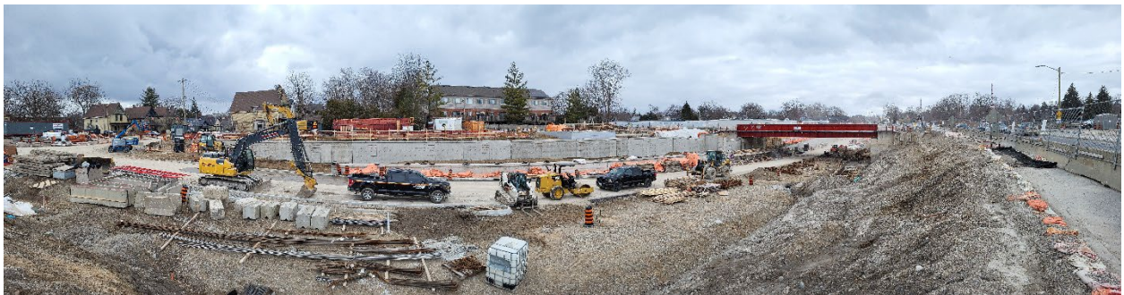
Above: Construction site for the Adelaide Street North Underpass project.
