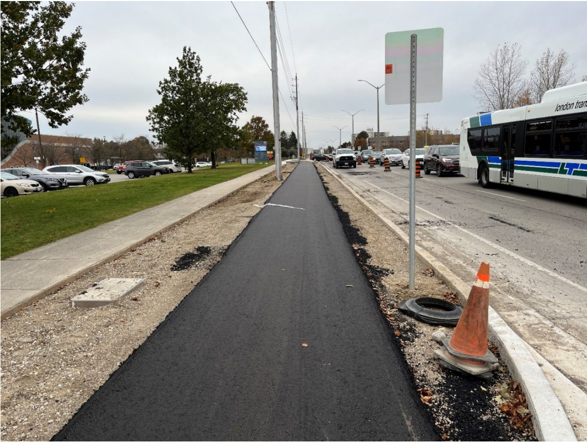
Above: A photo of the new in-boulevard bike lanes constructed in 2023 as part of the Bradley Avenue Cycle Track.
