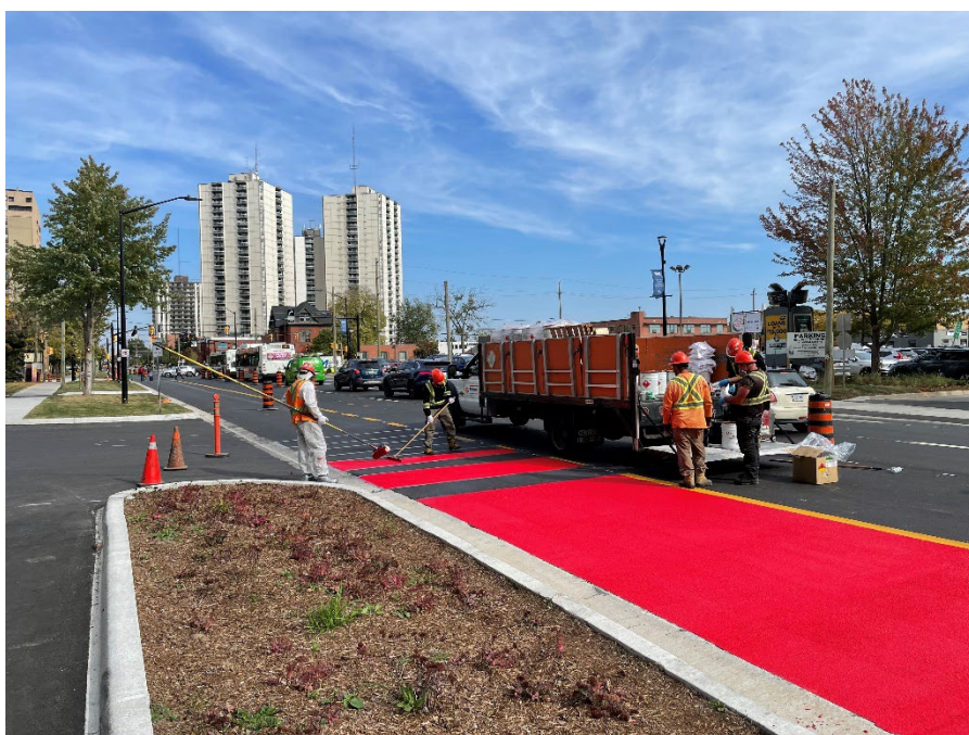
Above: Red paint operations at King Street.
