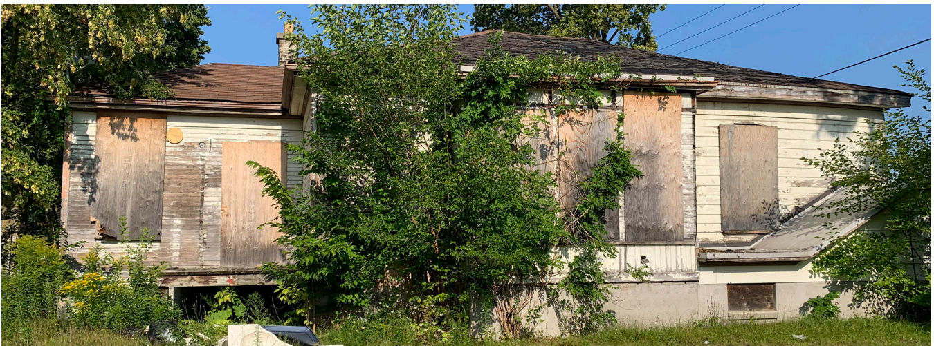
Photo 4.4: House on 520 South Street: view of west facade.
