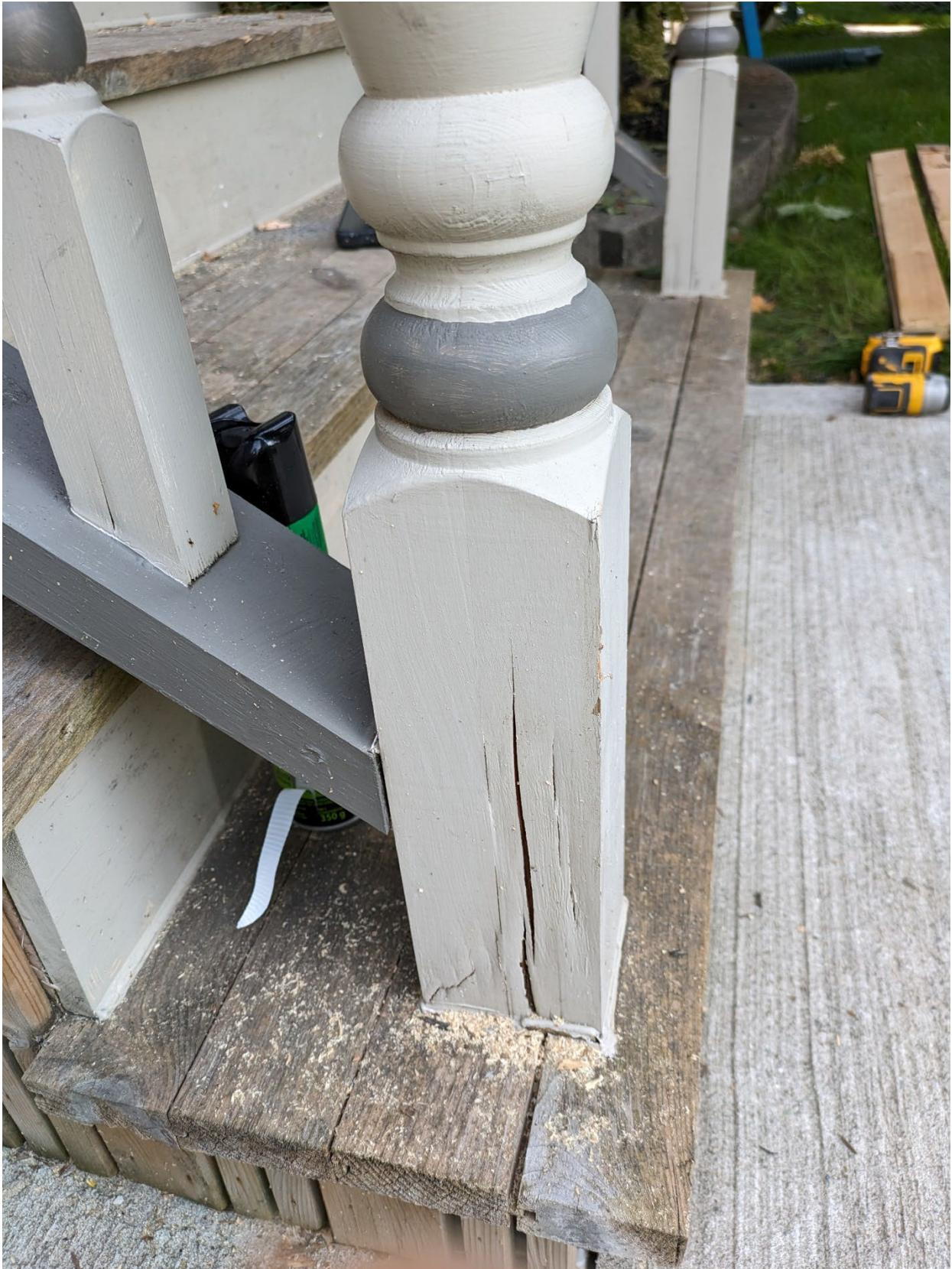
*Image 4: Photograph submitted with the Heritage Alteration Permit application demonstrating need for repair or replacement of the post on the front porch steps at 332 St James Street.*
