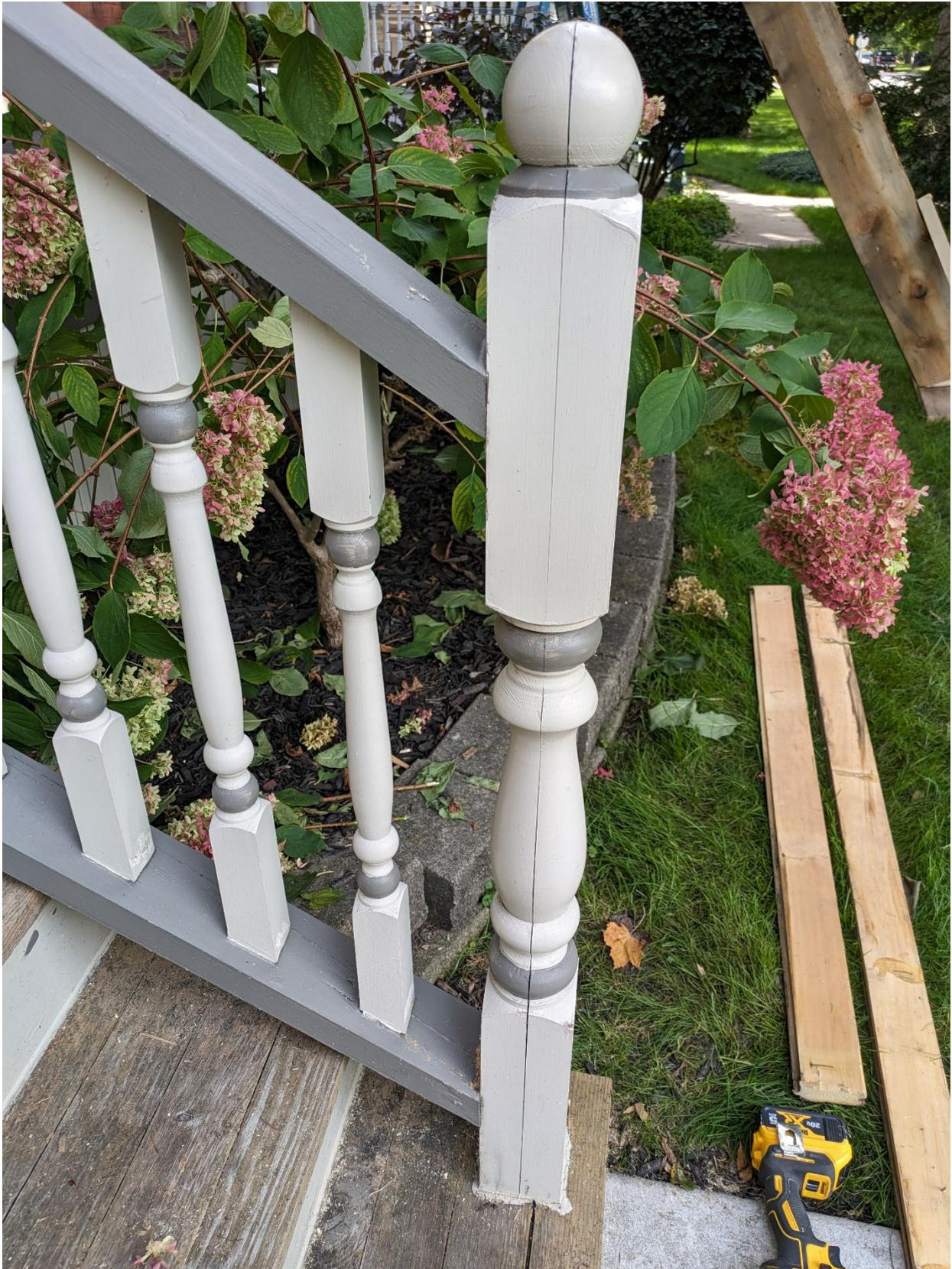
*Image 3: Photograph submitted with the Heritage Alteration Permit application demonstrating need for repair or replacement of the post on the front porch steps at 332 St James Street.*
